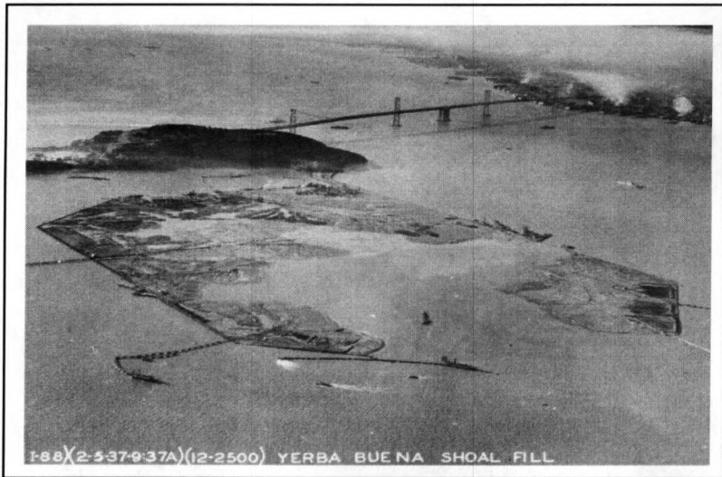
Figure 3. Filling of Yerba Buena Shoals, showing construction of the administration and hangar buildings, February 5, 1937. [Unit 2, Shelf B, Folder Treasure Island, Construction and Plans, Treasure Island Museum Collection]
