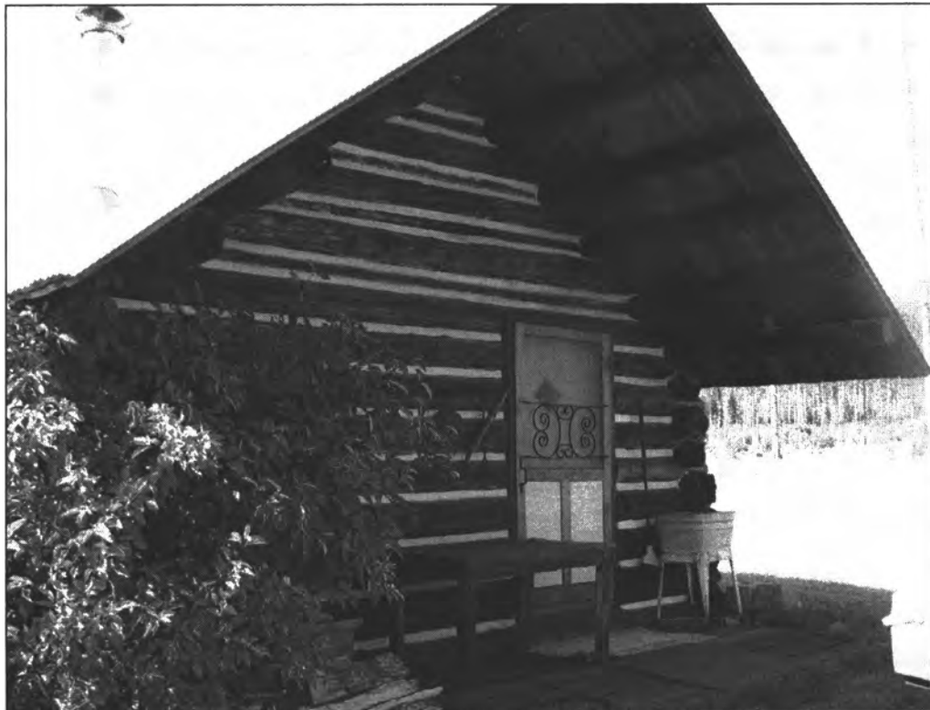
Photo 0003. Looking north-northwest; detail of the front (southeast) wall showing the overhang and board stoop.
