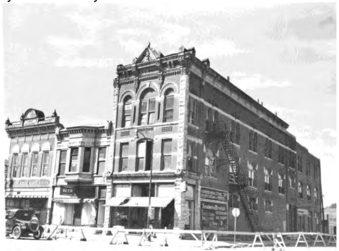
Figure 15—White/Clever and adjacent buildings at SW corner of 2 nd & Main (Buildings #28-27-26)
