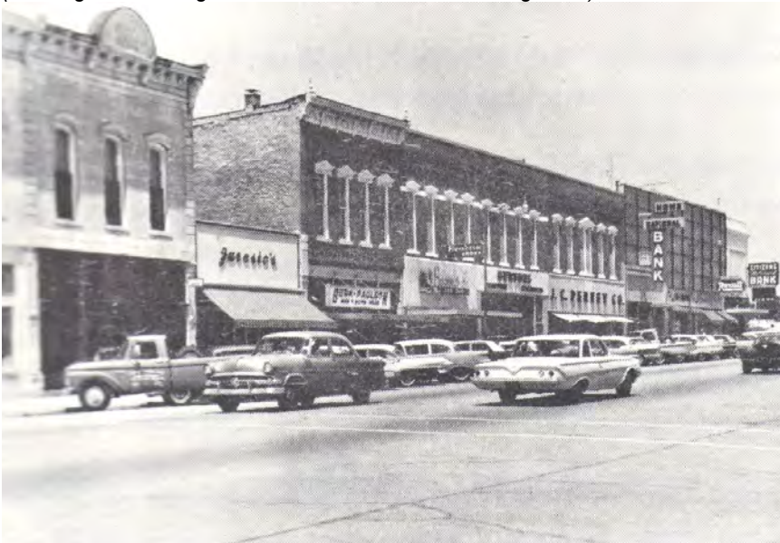
Figure 10 – ca. 1970s view of west side 200 block N. Main (Buildings #18-17-16-15-14-13-12-11-10)
