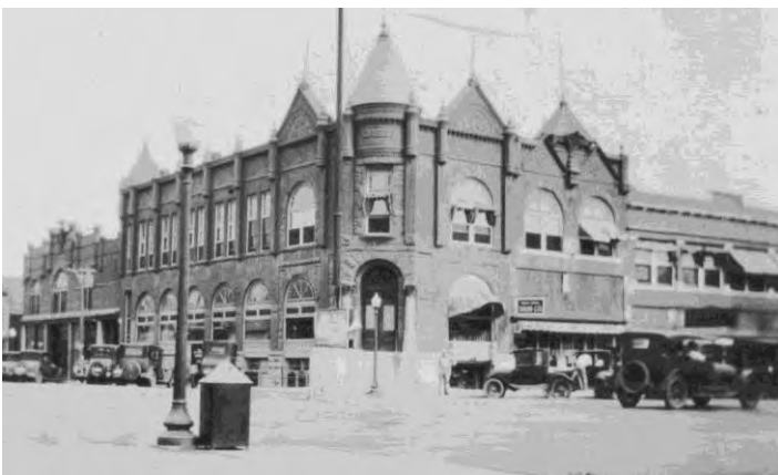
Figure 22—Farmers & Drovers Bank/Crebo Building (#63-62-61) at SE corner of 3 rd & Main
