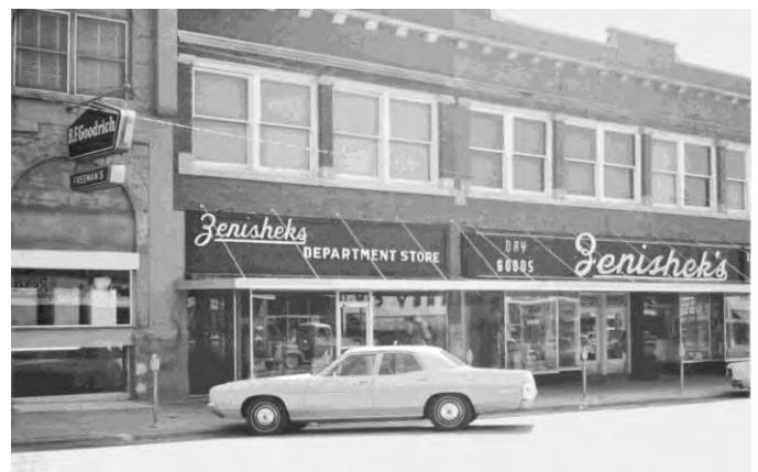
Figure 23—Crebo Building reconstructed after 1937 fire (#63-62-61)
