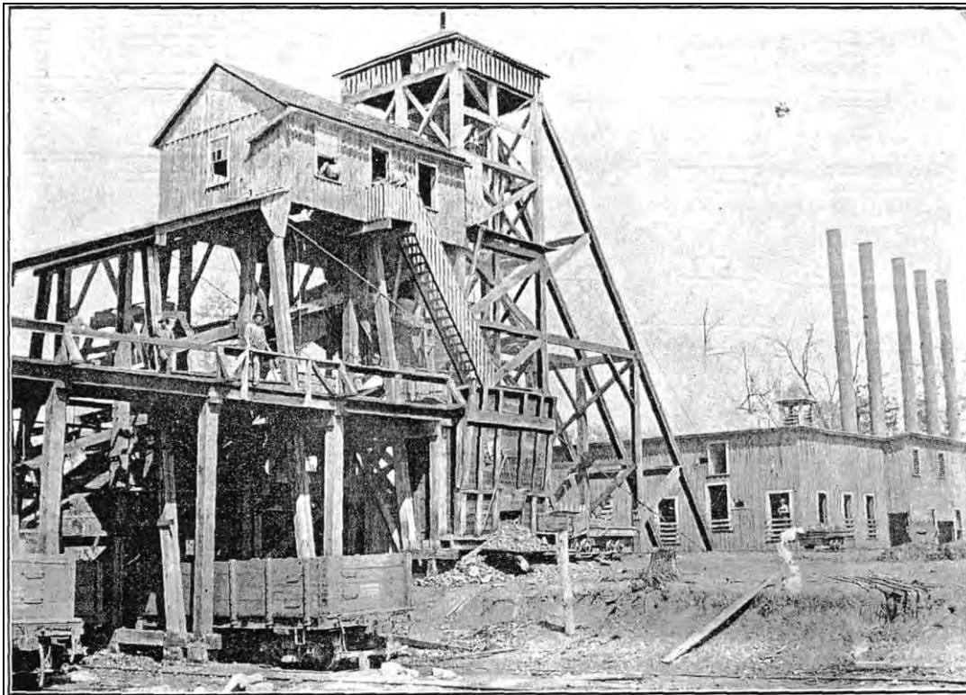
Figure 4: Tipple and Power Plant, Date Unknown, Photographer Unknown. Photo courtesy of Bon Air Historical Society.
