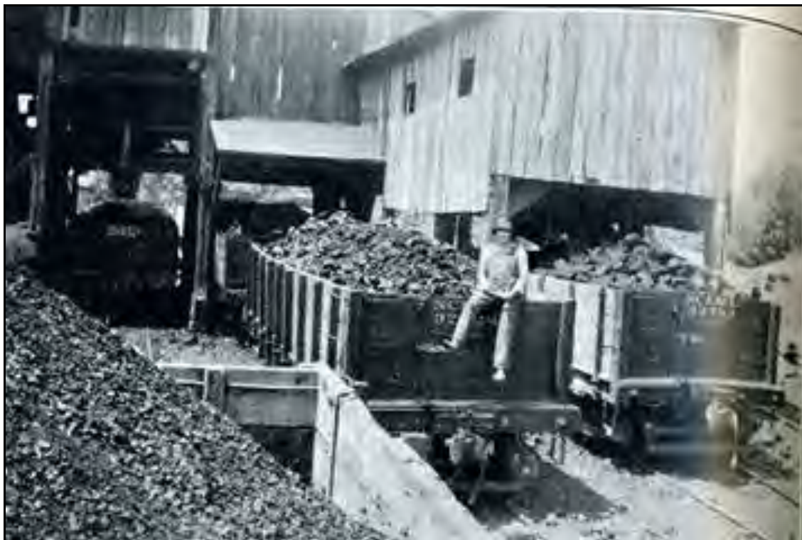
Figure 8: Loading three sizes of coal at Ravenscroft tippie, Tennessee Products Corporation. Photo courtesy of The Southern Tennessee Coal Field by Wilbur Armistead Nelson.
