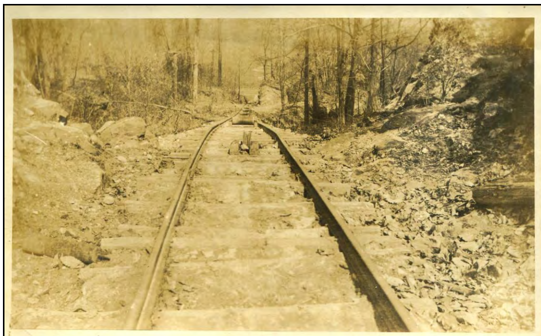
Figure 28: Ravenscroft Rail bed, c. 1921. Photo courtesy of Bon Air Historical Society.
