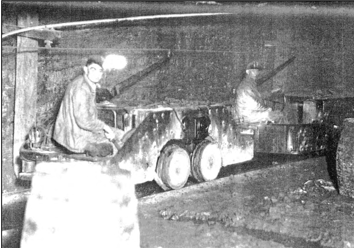
Figure 15: Motors at Shaft Bottom in Ravenscroft Mine, Tennessee Products Corporation. Date Unknown, Photographer Unknown. Photo courtesy of The Southern Tennessee Coal Field by Wilbur Armistead Nelson.
