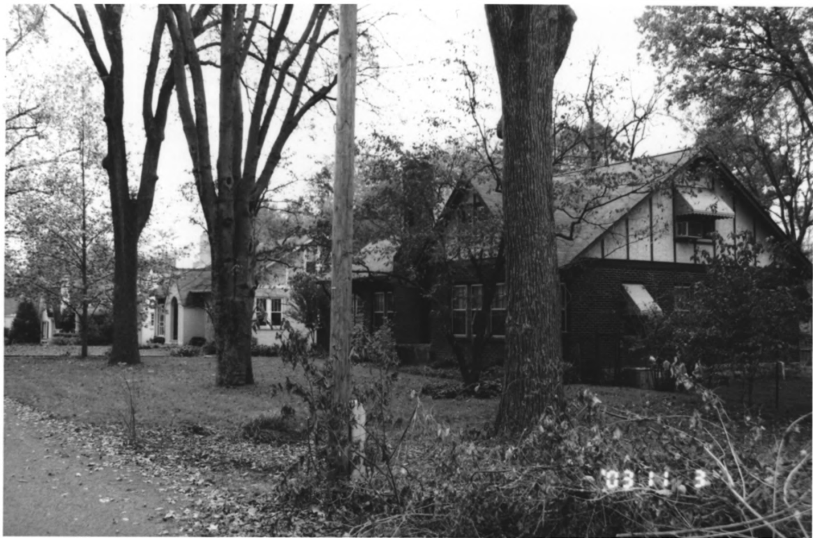
Belle Meade Golf Links Subdivision Historic District '14 Davidson County TN
