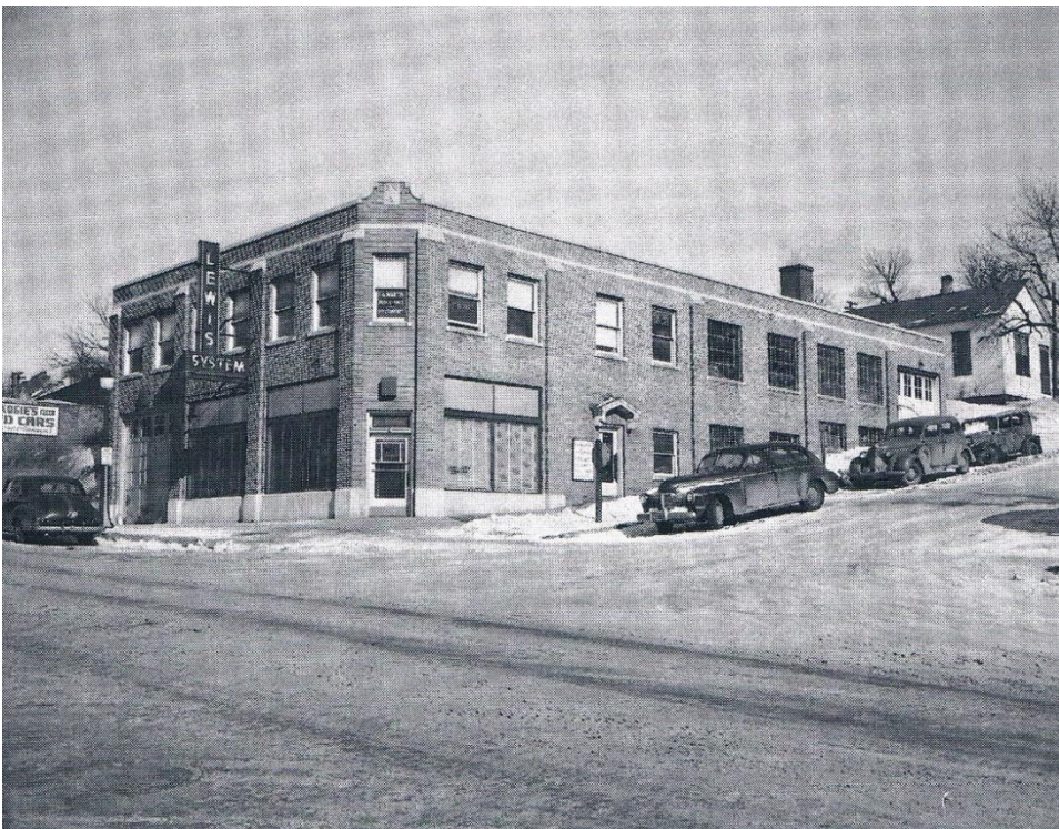
PHOTO 5: Lewis System building, c. 1945. Image courtesy of Sioux City Public Museum Research Center, December 2014.
