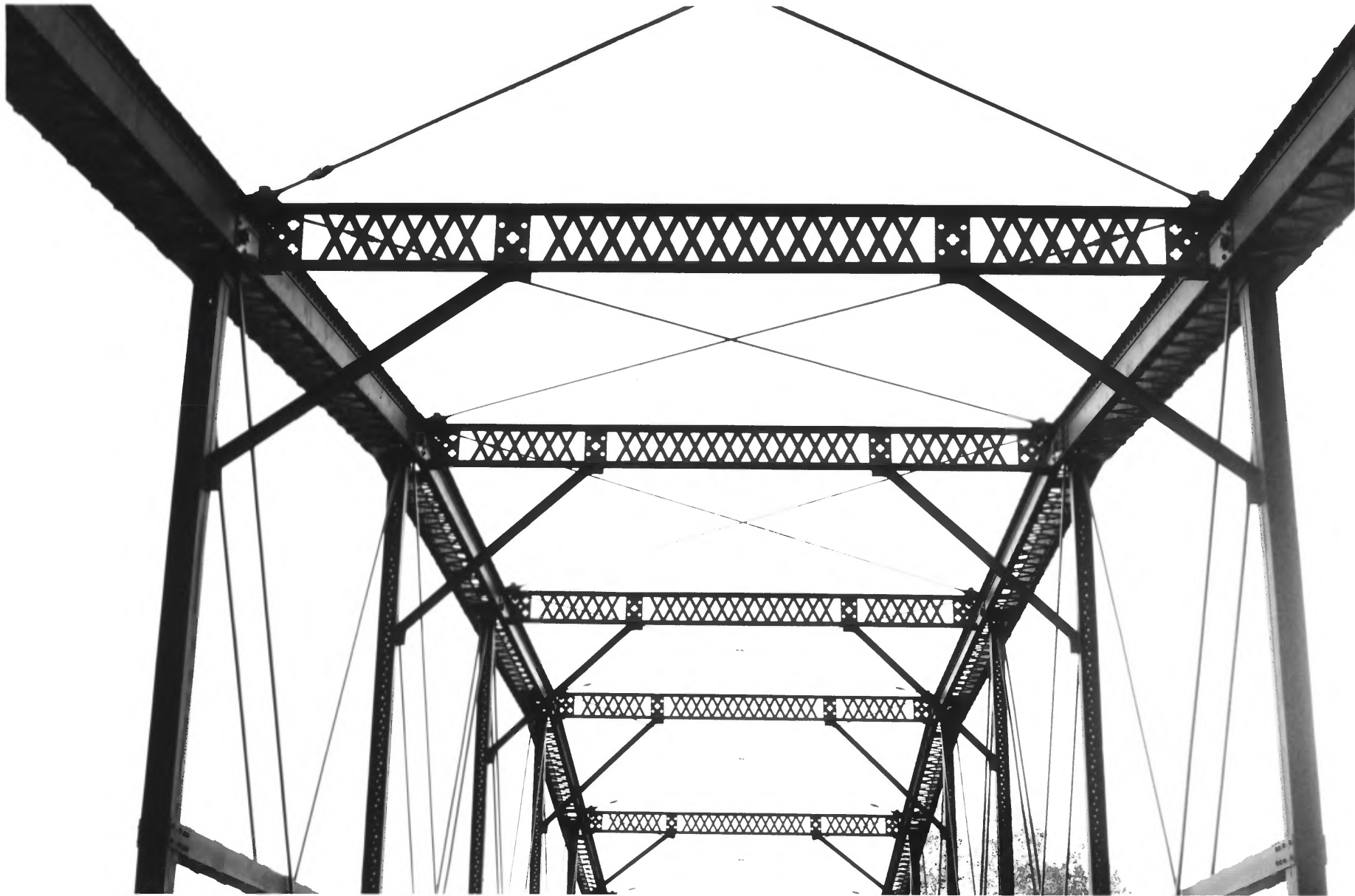
Bridge no. 5721 mn Highway 65 over Little Fork River, Unorganized Territory (Vicinity of Rauch) Koochiching Co., mn 012622-11A/12
