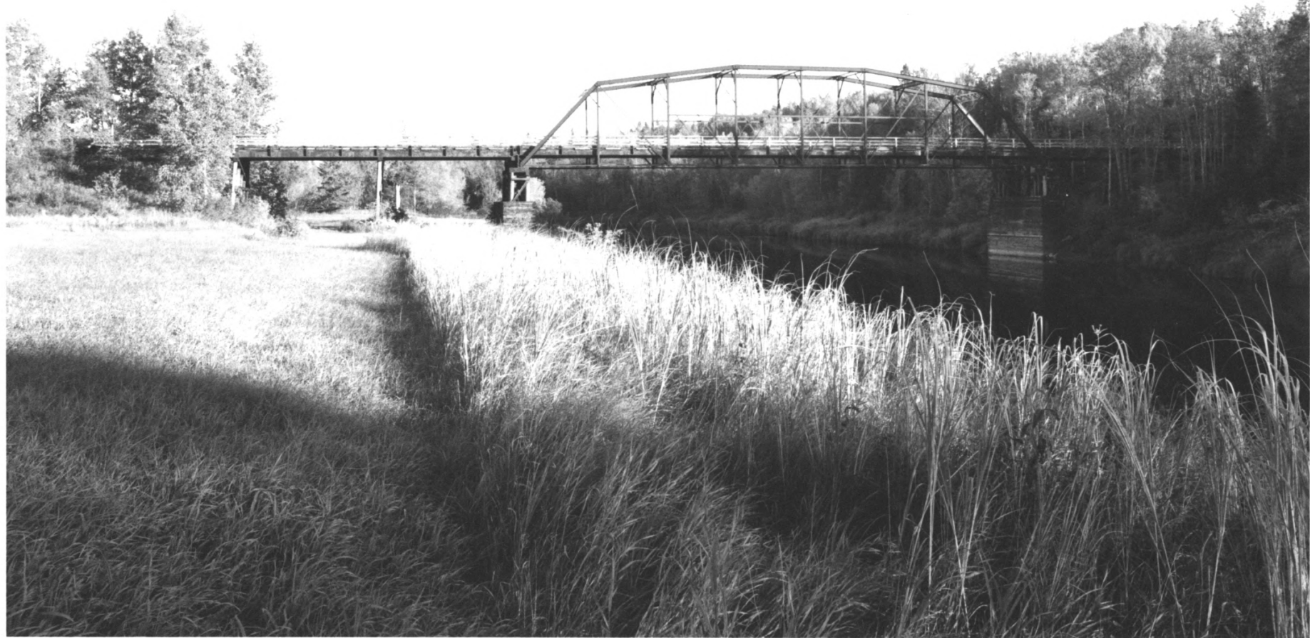
Bridge no. 5721 Mn Highway 65 over Little Fork River, Unorganized Territory (Vicinity of Rauch) Koochiching Co., Mn 012616-23
