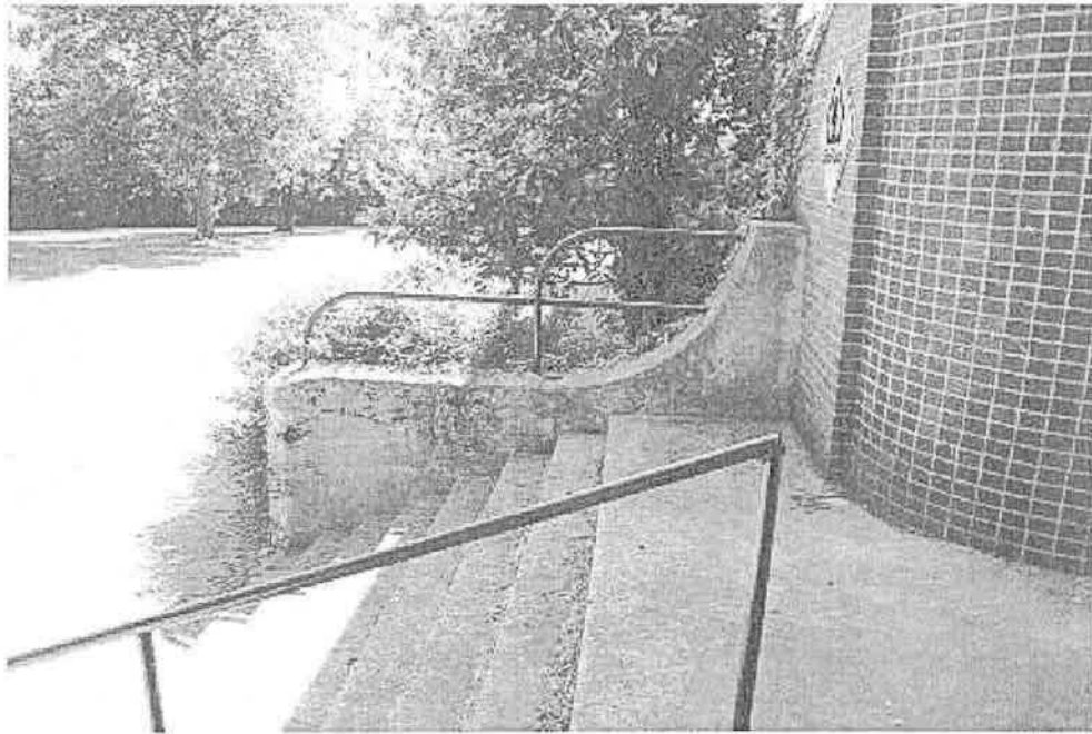
Figure 9: Curved concrete forms, handrails, and brick walls.
