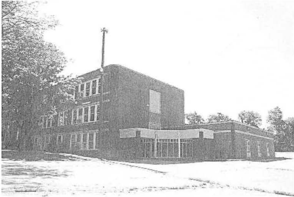
Figure 11: West side addition
