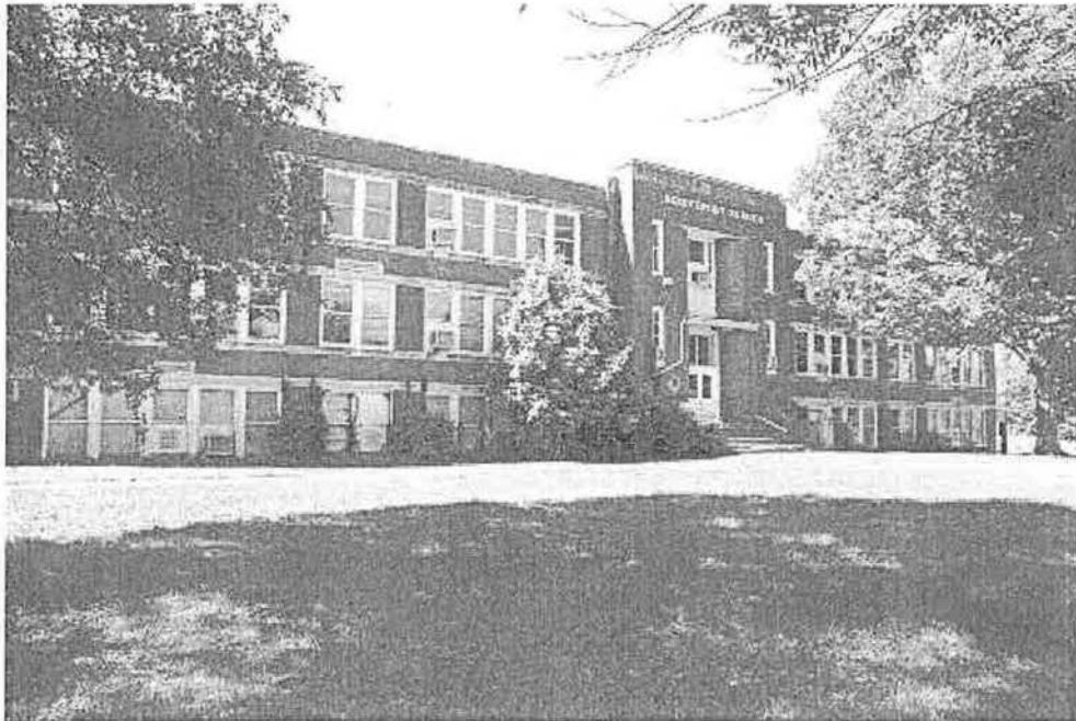
Figure 1: View of front elevation
