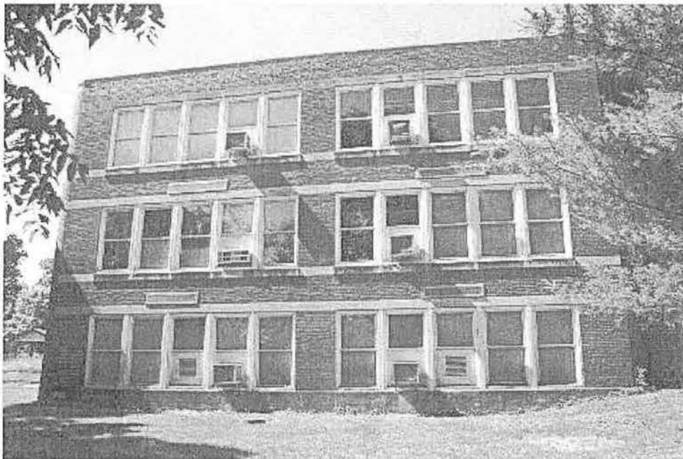
Figure 3: Offset wing of the building
