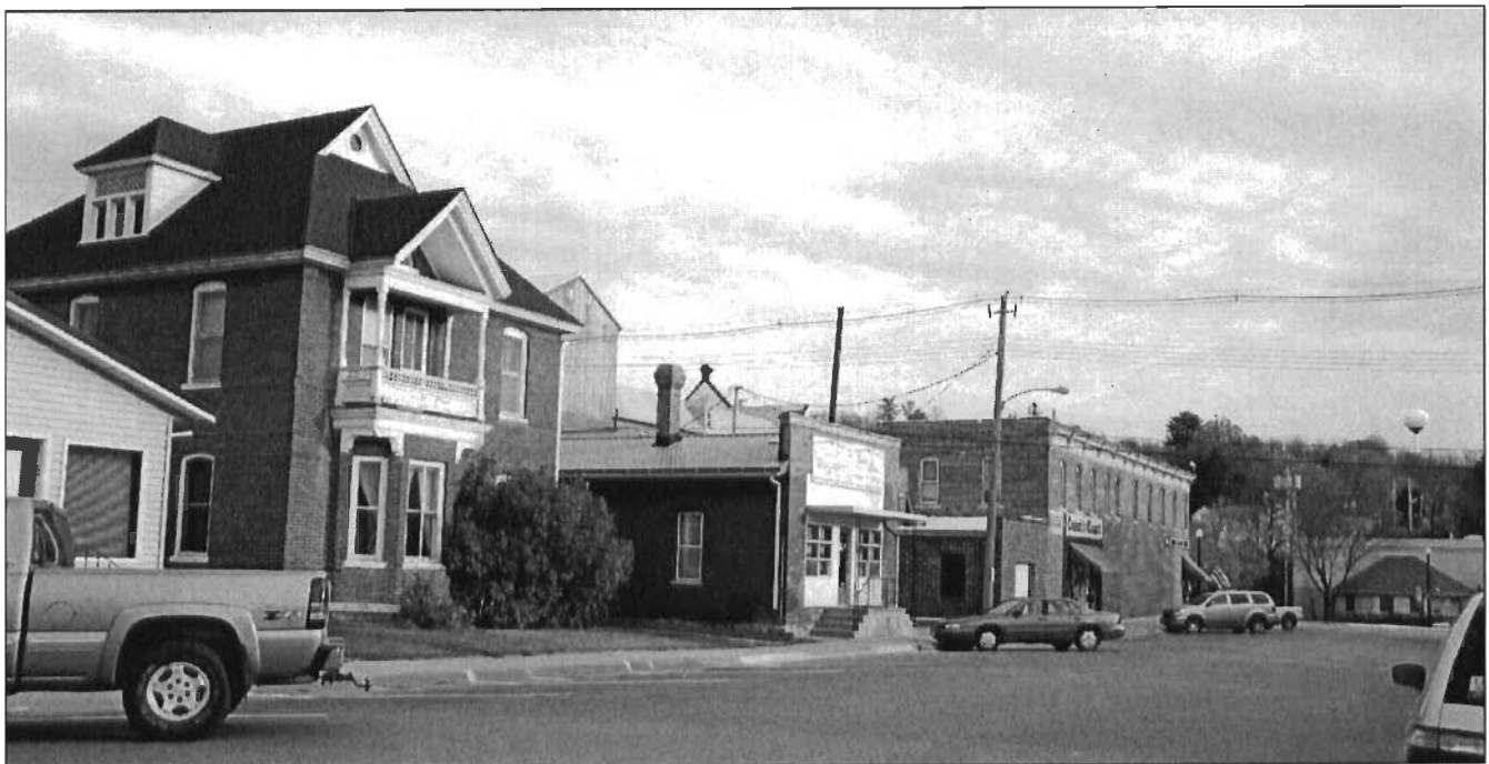
Photograph 24: Street view of north side of 100 block of West Cedar Street, looking east from First Street (9/16/2010, Marlys Svendsen, photographer)
