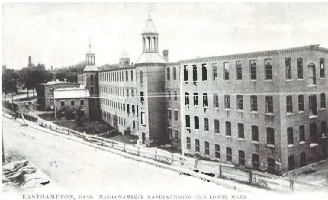
Fig. 2. Postcard view ca. 1905. Facing northwest across Cottage Street towards Buildings 8,9, 10, 15 and 21
