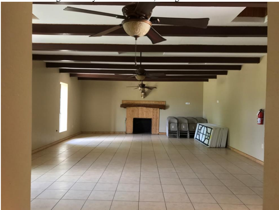
Photo 14 East room through doorway from west room, facing east
