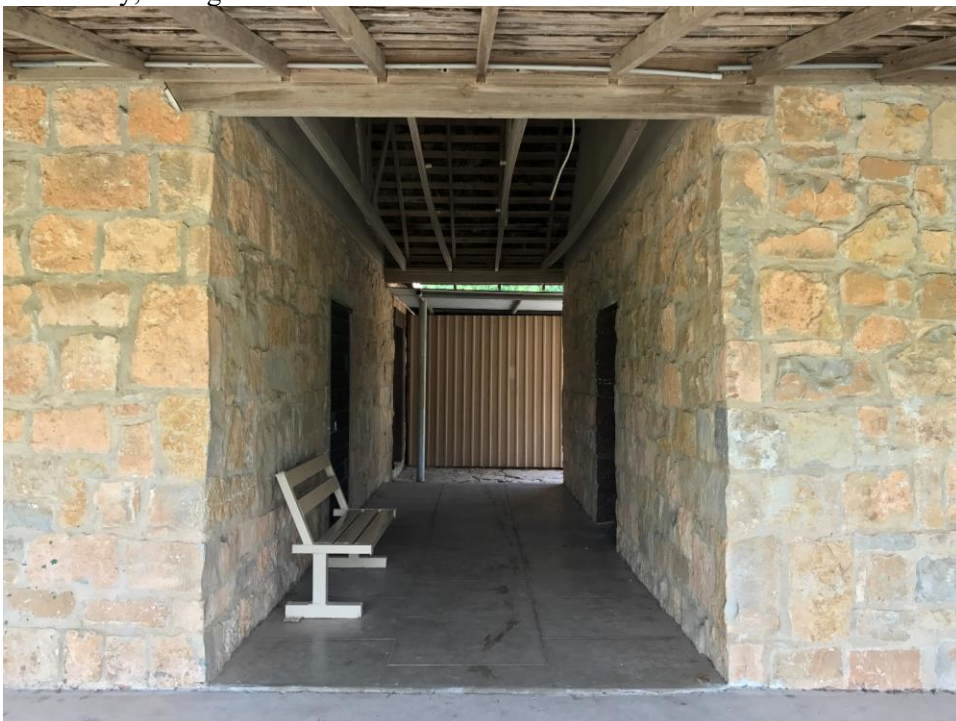
Photo 10 Breezeway, facing east towards addition
