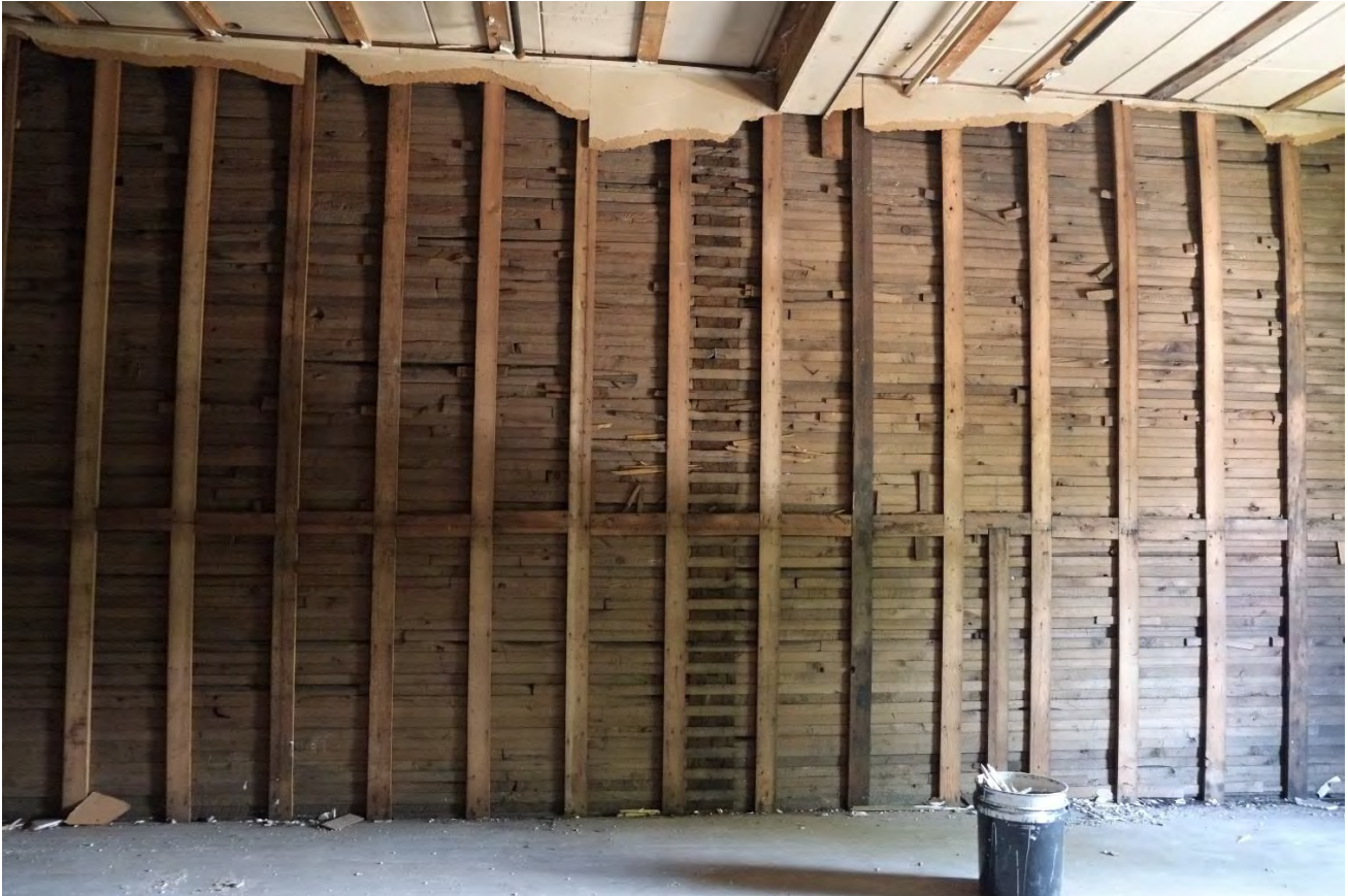
Figure 2: Crib construction inside Malt House grain elevator
