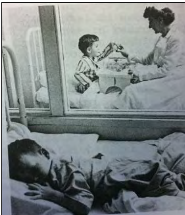
Figure 16: Infirmary showing glass walls. Source: Helen Schick Lane. "History of CID," 1981, p. 30. Date unknown.
