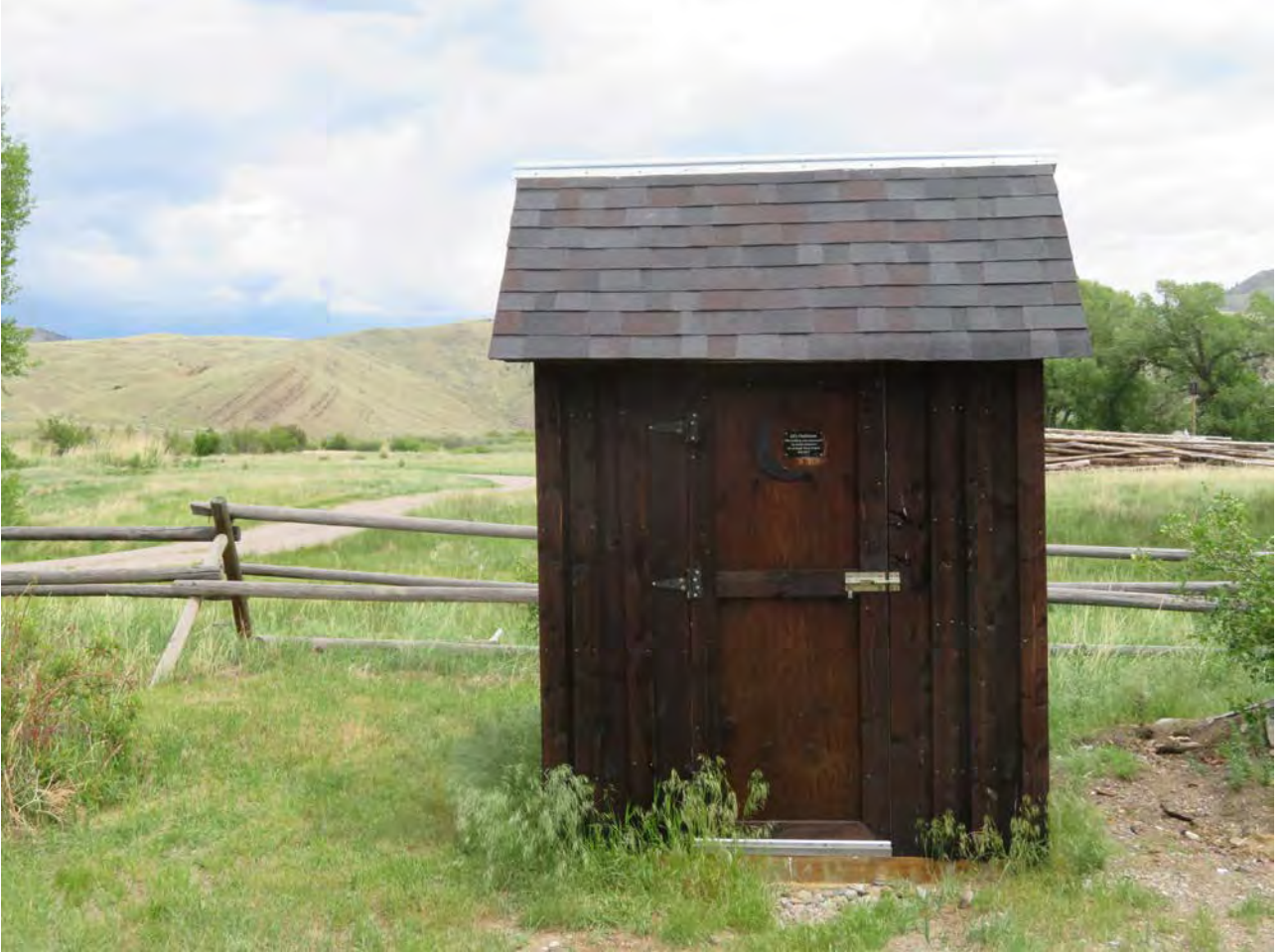
Photo 0026. Solar Battery Bank House. View to north.
