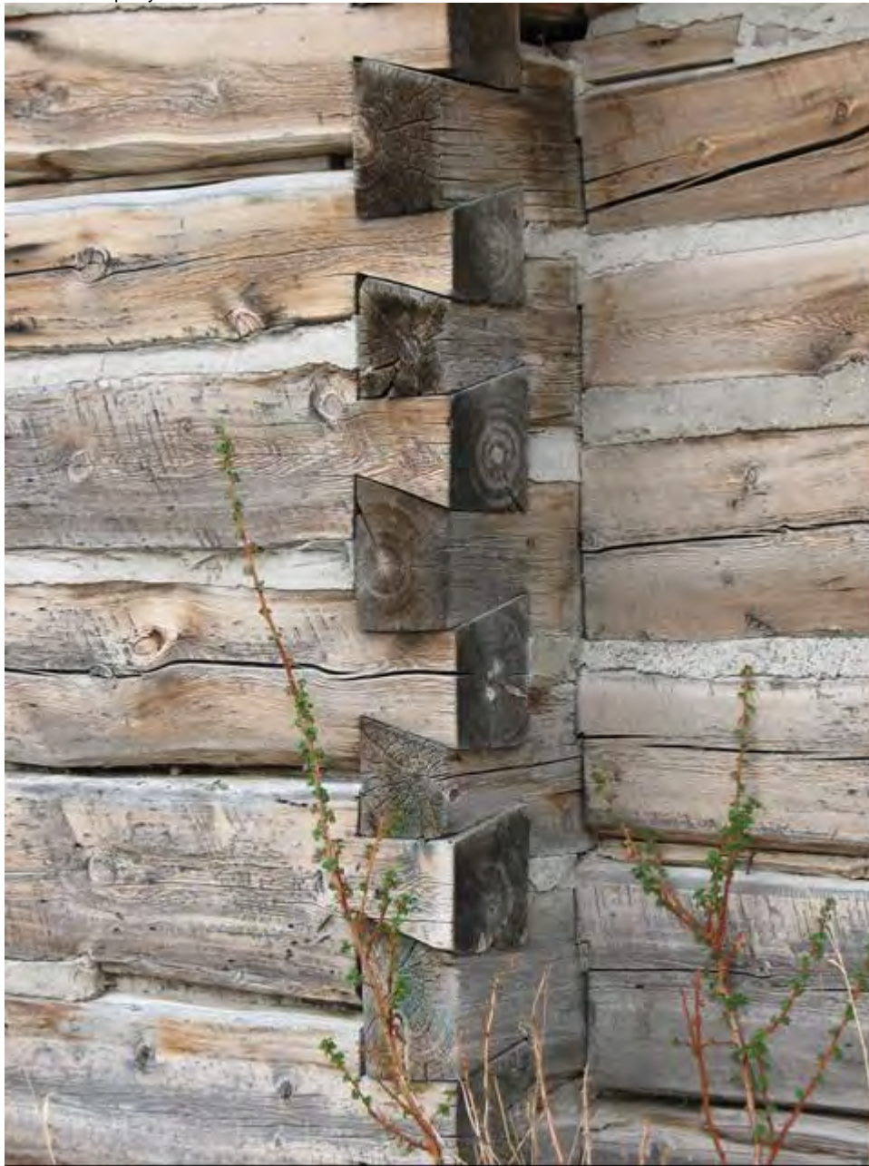
Photo 0007. 1905 House (C), notching detail at north central corner. View to southeast.
