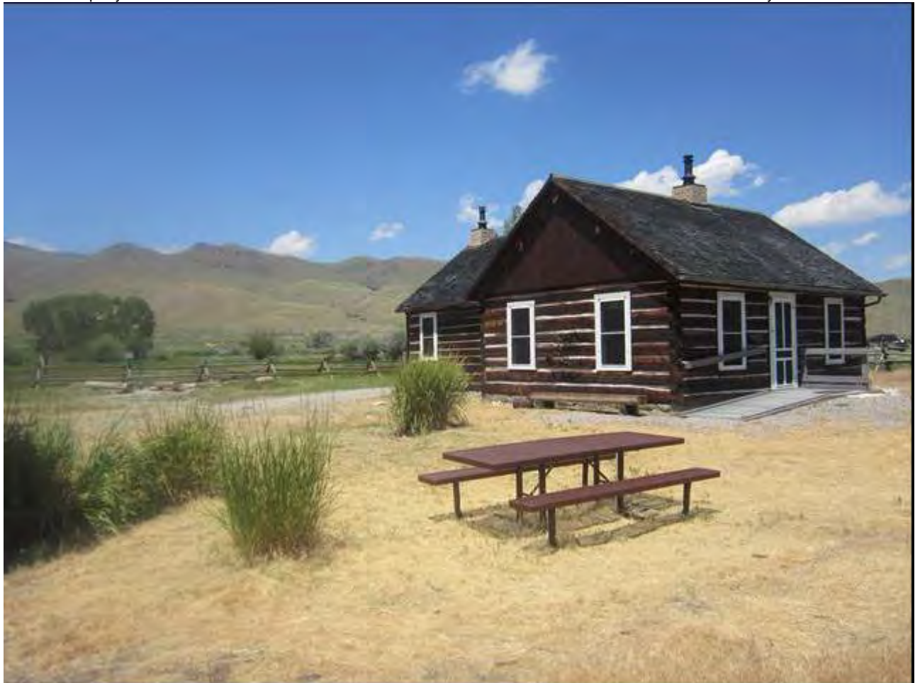
Photo 0005. 1905 House (C), south and east elevations. View to northwest.
