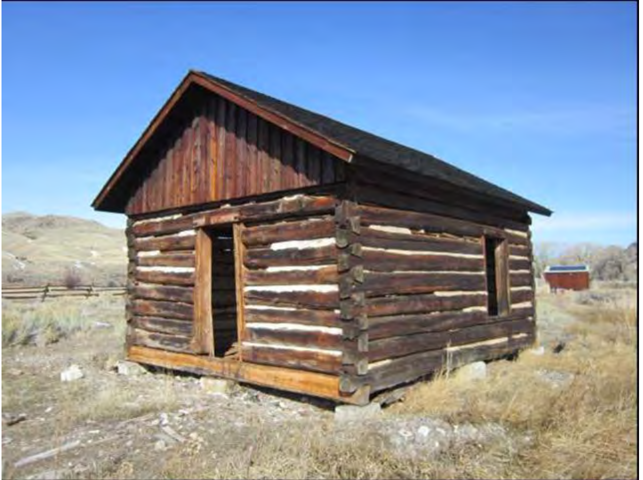
Photo 0008. 1883 Cabin (A), south and east elevations, View to northwest.
