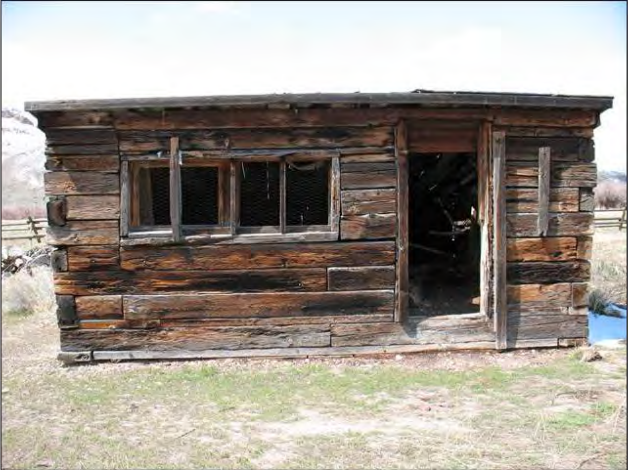
Photo 0010. Chicken Coop (B), east elevation. View to west.
