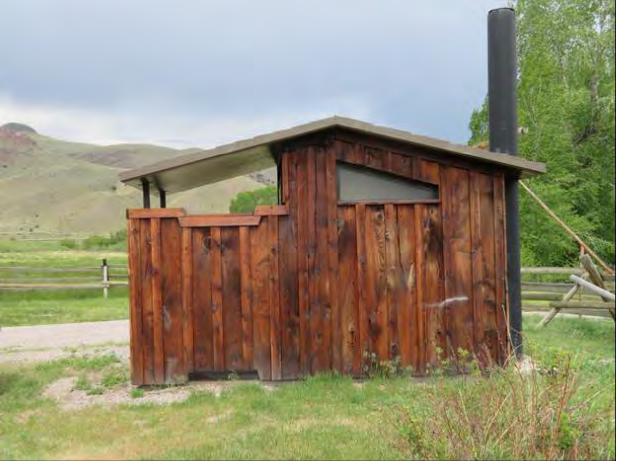
Photo 0024. Vault Toilet. View to west.
