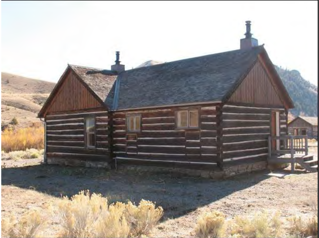
Photo 0004. 1905 House (C), north and west elevations. View to southeast.
