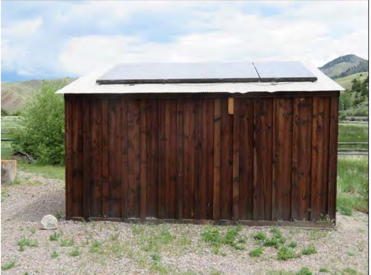
Photo 0028. Wood Shed with Solar Panels. View to north.
