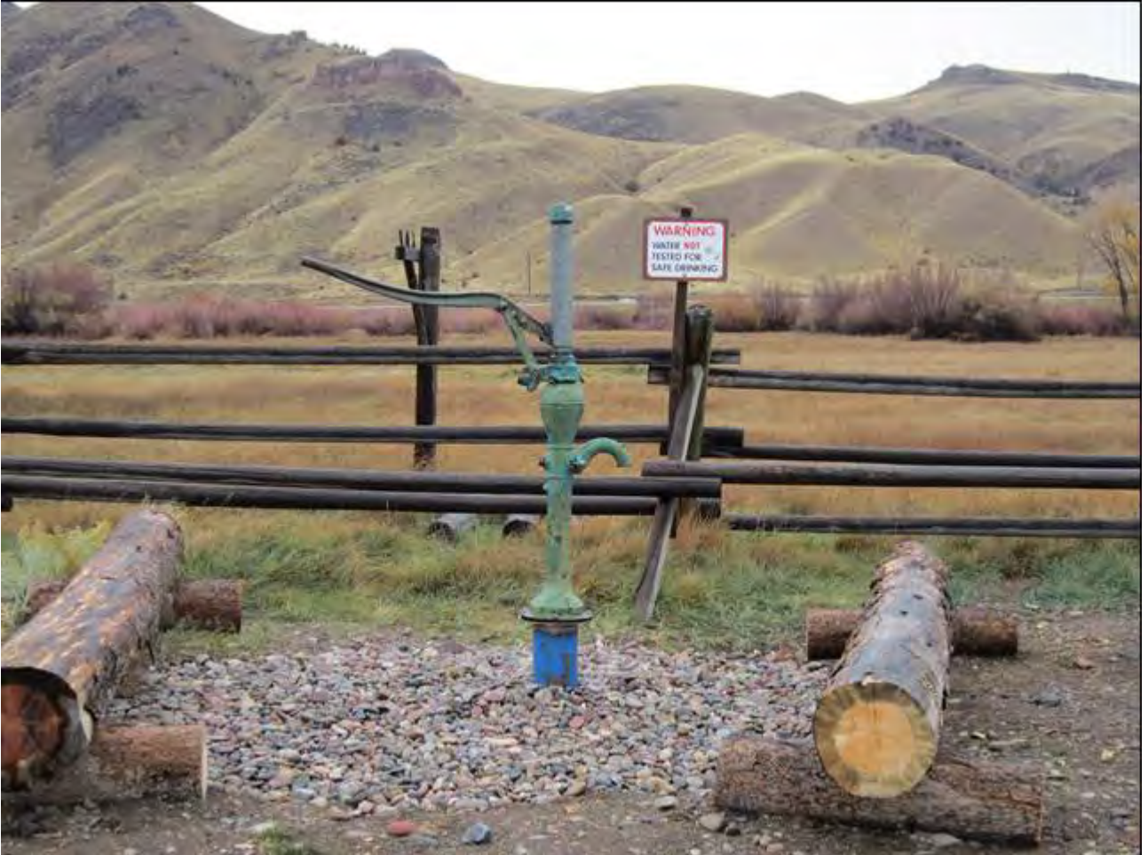
Photo 0025. Well and Pump. View to west.
