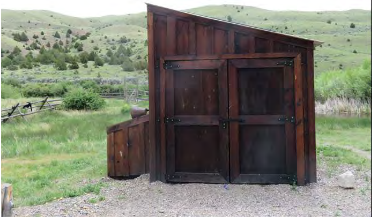
Photo 0027. Wood Shed. View to east.
