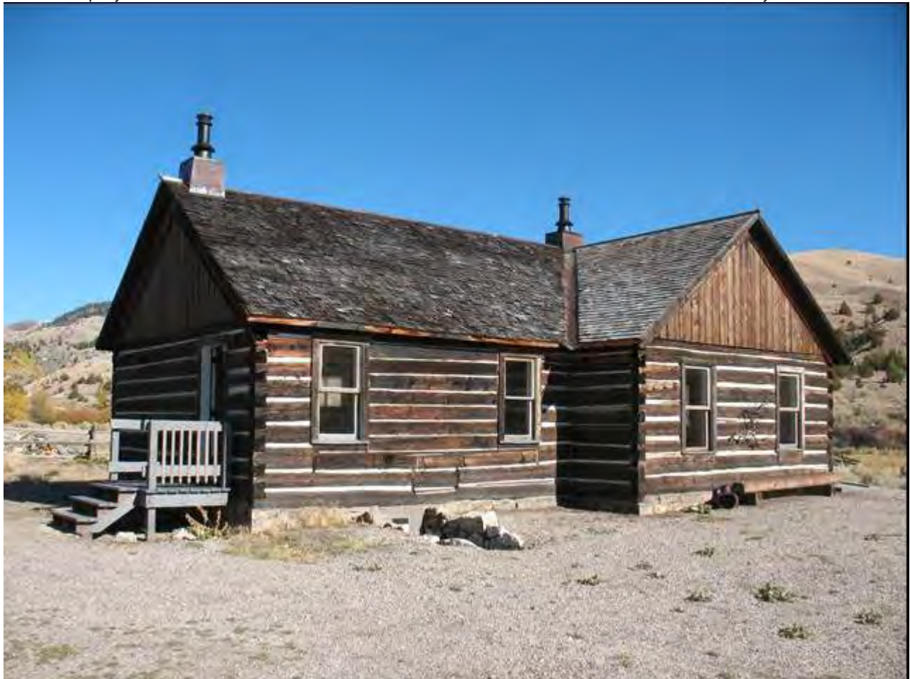
Photo 0003. 1905 House (C), south and west elevations. View to northeast.
