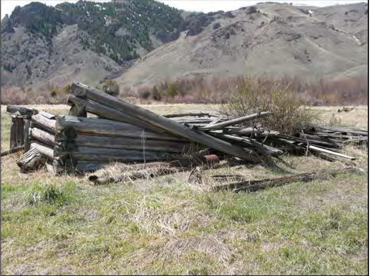
Photo 0012. Possible Barn (D), north and east elevations. View to southwest.
