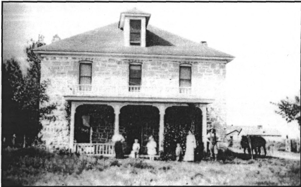
Figure 2. This photograph of the ranch house was taken around 1903 and shows the original design of the front entry porch, with painted turned wood columns and decorative balusters. (Photo from Four Score for Dave Hamil by Bud Wells)
