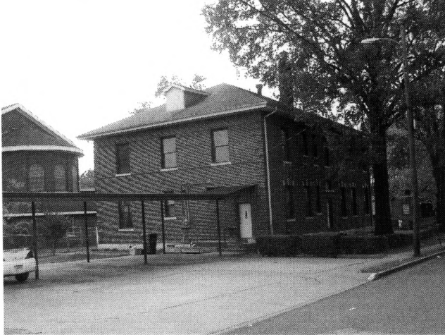
East and north facades of convent.
