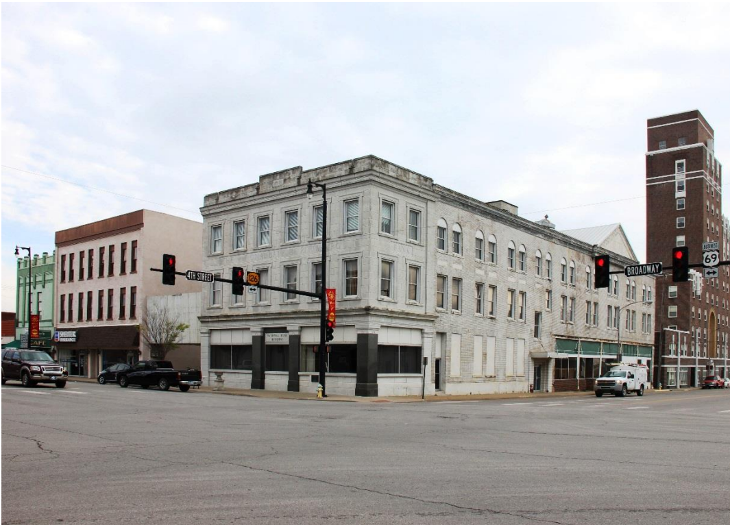
2 of 17: Left to Right: 412 and 408-410 N. Broadway, 105 and 121 E. 4 th Street. Camera facing northeast.
