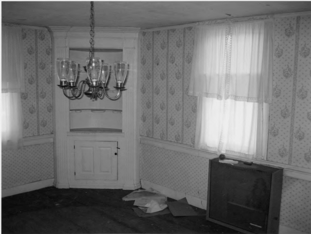
The Elam Ives House Hamden, New Haven County, Connecticut Photograph 6 The corner cupboard in the northeast room April 2007 James Sexton
