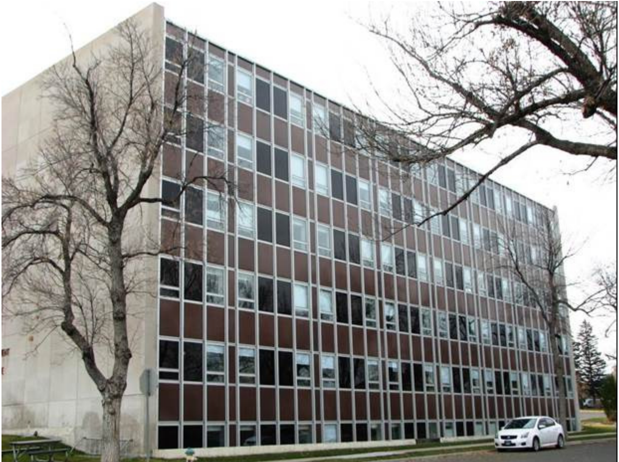
1956 Addition to the Montana Highway Department Building (Scott Hart Building) North Elevation, Facing: SW Montana State Capitol Campus Historic District Helena, Lewis & Clark County, Montana Jessie Nunn, October 25, 2014 MT_MontanaStateCapitolCampusHD_0011
