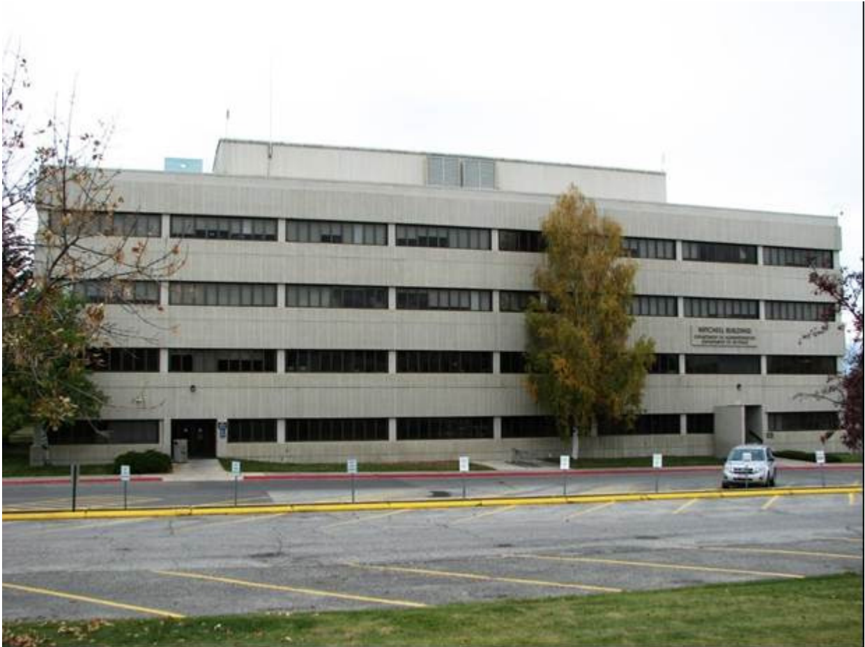
1975 Addition the State Office Building (Sam W. Mitchell Building) East Façade, Facing: SW Montana State Capitol Campus Historic District Helena, Lewis & Clark County, Montana Jessie Nunn, October 11, 2014 MT_MontanaStateCapitolCampusHD_0013
