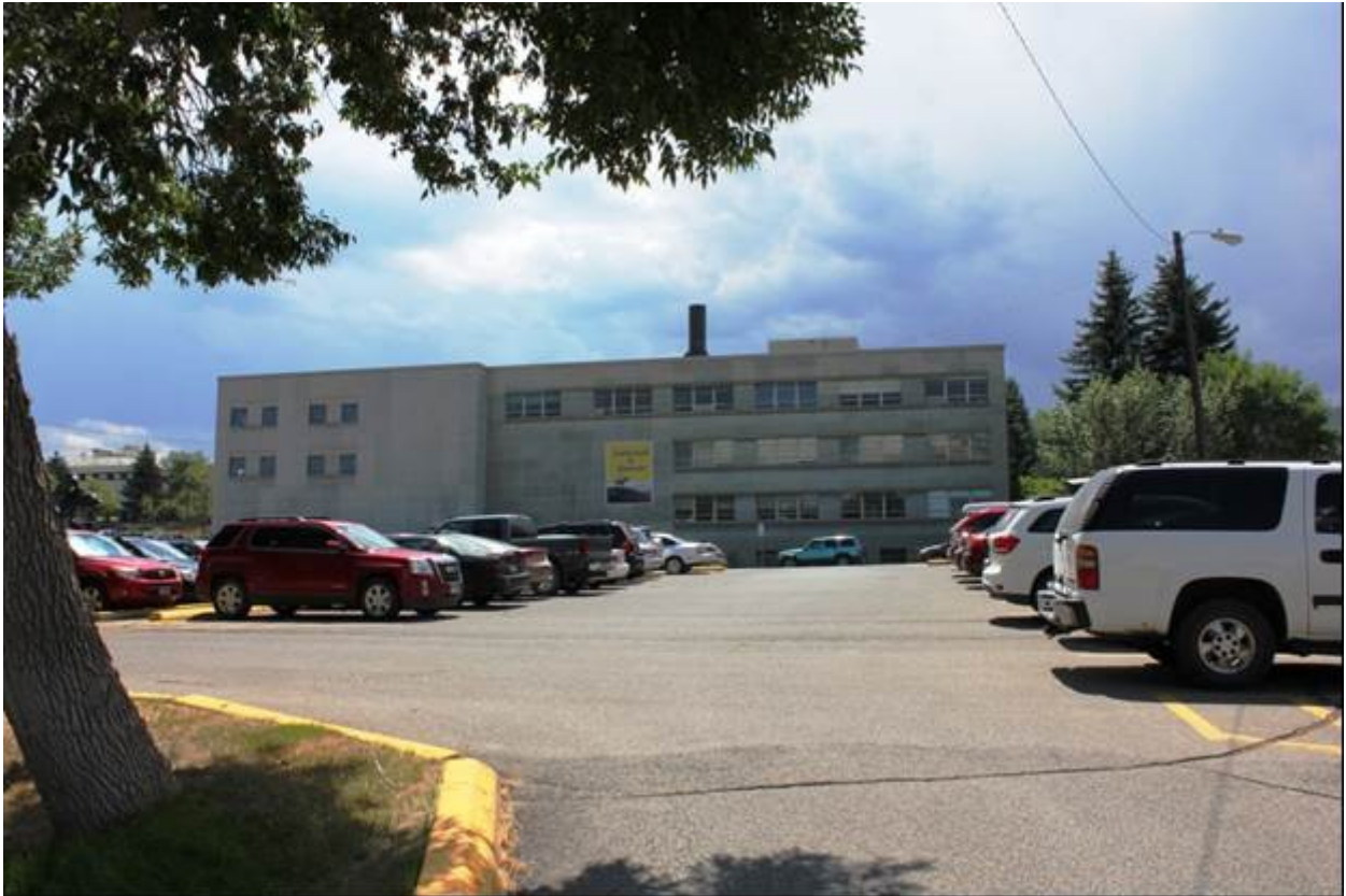
Montana Veterans & Pioneers Memorial Building North Elevation, Facing: S Montana State Capitol Campus Historic District Helena, Lewis & Clark County, Montana Kate Hampton, June 22, 2015 MT_MontanaStateCapitolCampusHD_0018
