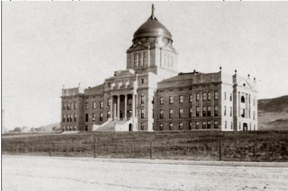
Montana State Capitol, Architectural Drawing by Bell & Kent, c. 1898 (Above). Montana State Capitol, c. 1904 (Below). (Helena As She Was Website, "Views of the Capitol").
