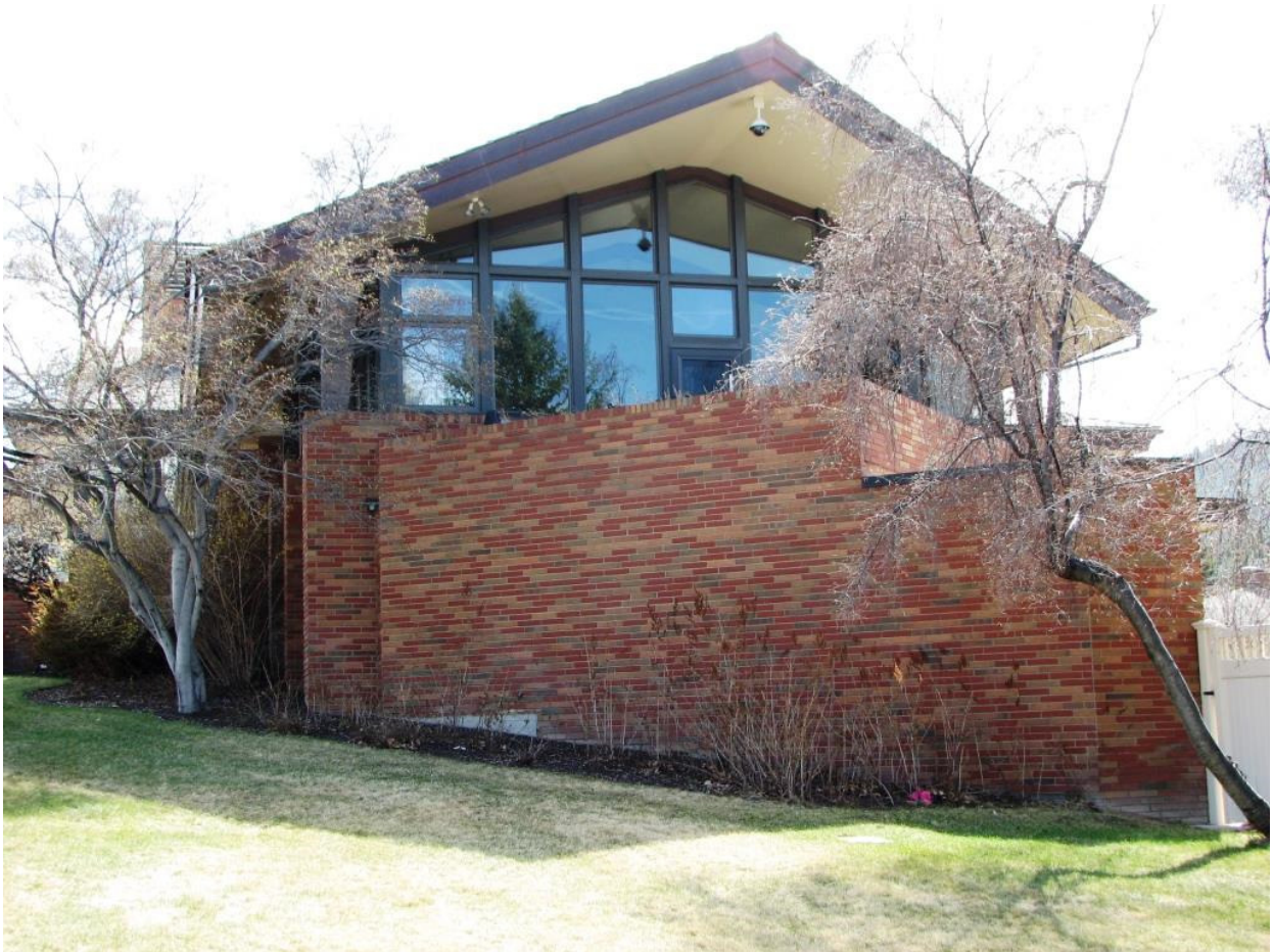
Governor's Mansion / Executive Residence North Elevation, Facing: SW Montana State Capitol Campus Historic District Helena, Lewis & Clark County, Montana Jessie Nunn, April 10, 2015 MT_MontanaStateCapitolCampusHD_0021
