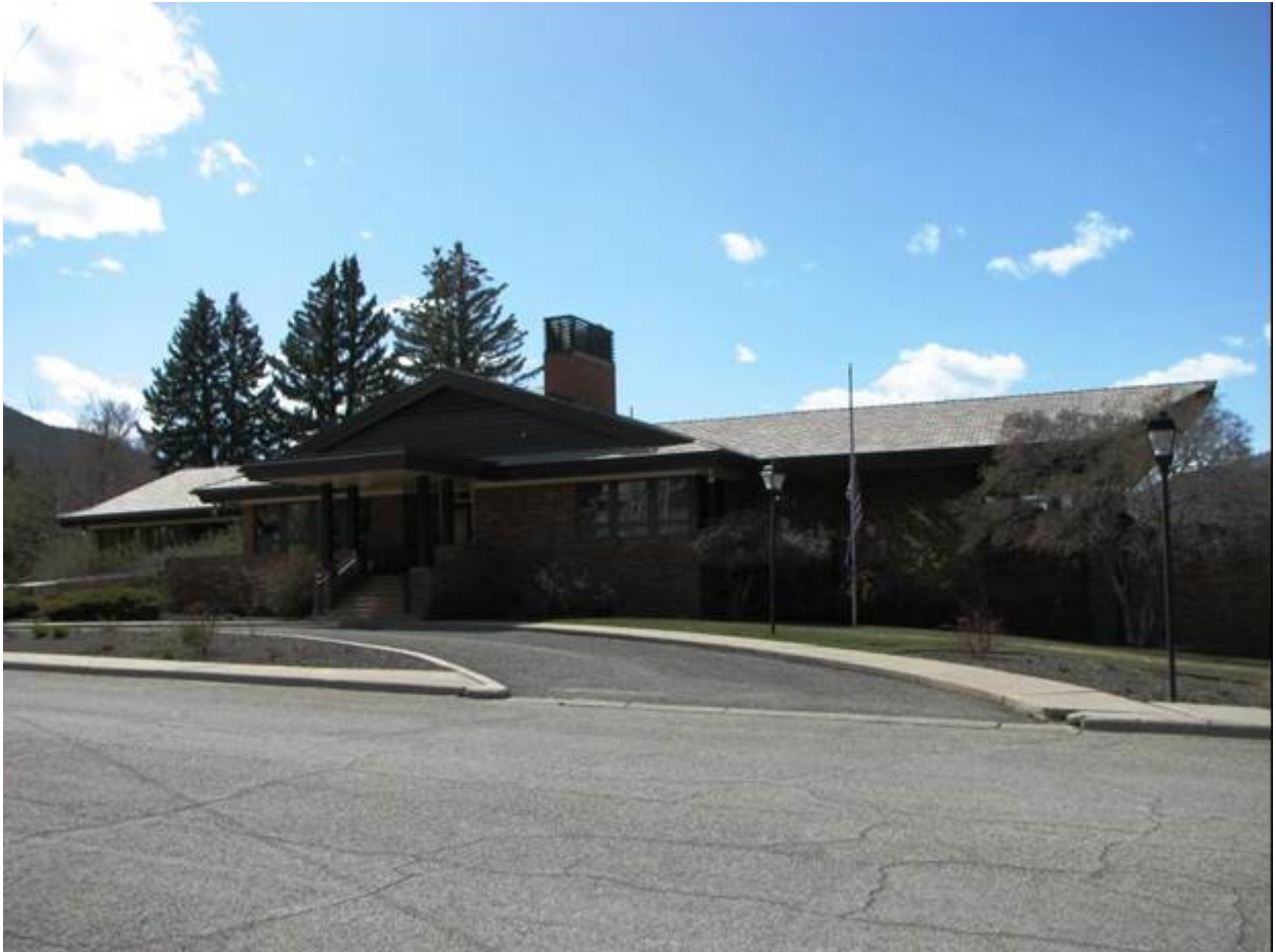
Governor's Mansion / Executive Residence East Façade, Facing: SW Montana State Capitol Campus Historic District Helena, Lewis & Clark County, Montana Jessie Nunn, April 10, 2015 MT_MontanaStateCapitolCampusHD_0019
