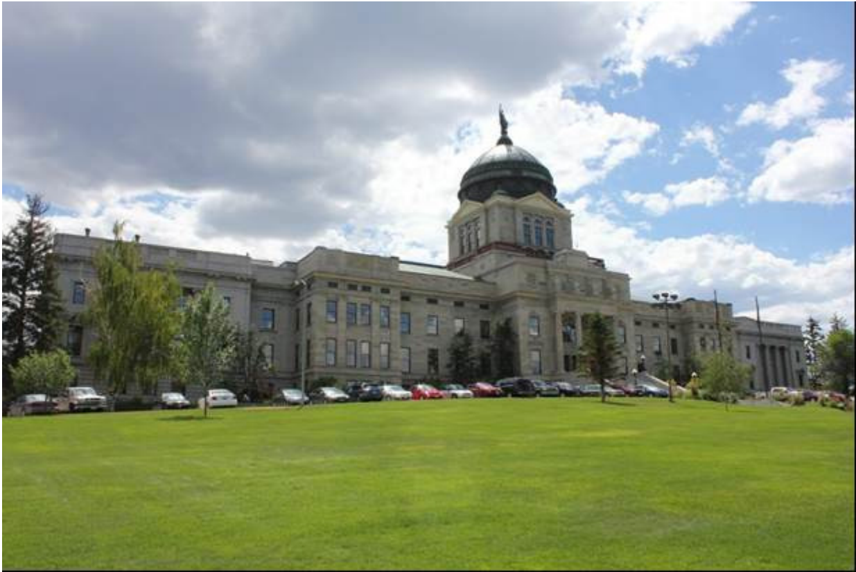
Montana State Capitol North Façade, Facing: SW Montana State Capitol Campus Historic District Helena, Lewis & Clark County, Montana Kate Hampton, June 22, 2015 MT_MontanaStateCapitolCampusHD_0001
