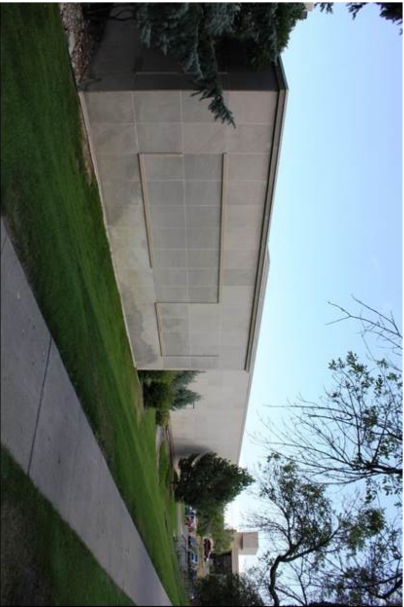
Montana Veterans & Pioneers Memorial Building South Elevation, Facing: NE Montana State Capitol Campus Historic District Helena, Lewis & Clark County, Montana Kate Hampton, June 22, 2015 MT_MontanaStateCapitolCampusHD_0017
