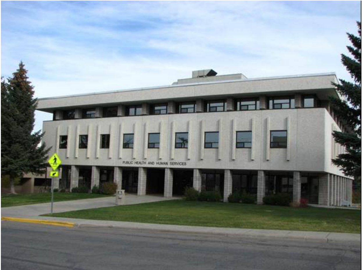
Social & Rehabilitation Services Building (DPHHS Building) West Façade, Facing: SE Montana State Capitol Campus Historic District Helena, Lewis & Clark County, Montana Jessie Nunn, October 25, 2014 MT_MontanaStateCapitolCampusHD_0027
