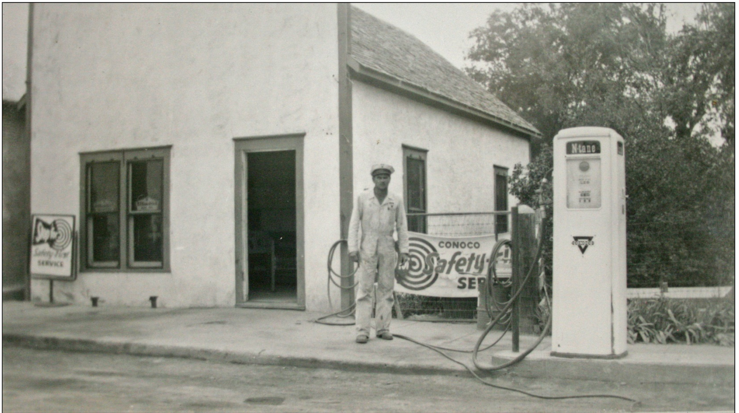
Figure 5. The false front building at the northeast corner of the property is shown in this undated (ca. 1950s) view southeast. Note the pump island featuring Conoco N-tane gasoline and the woven wire fence around the yard. Courtesy James and Clea (Covalt) Englehardt, photograph and clipping collection.
