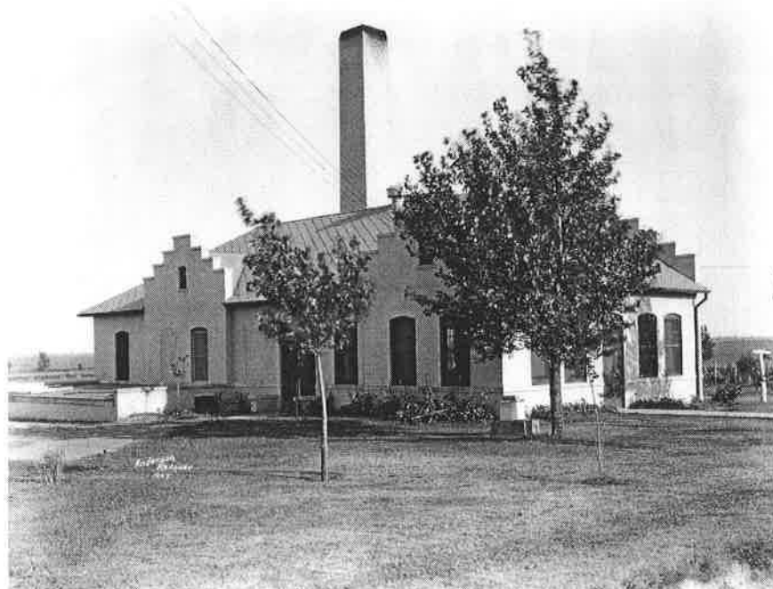
Figure 17: Laundry, north and west facades, 1927- A.T. Anderson/Kearney
