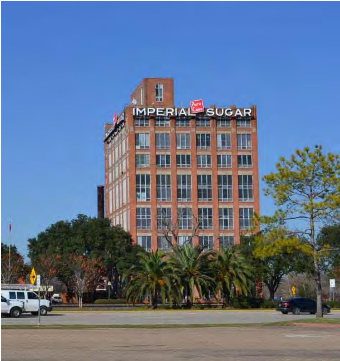
Photo 7 – Char House (Resource ID 1), south elevation, view north
