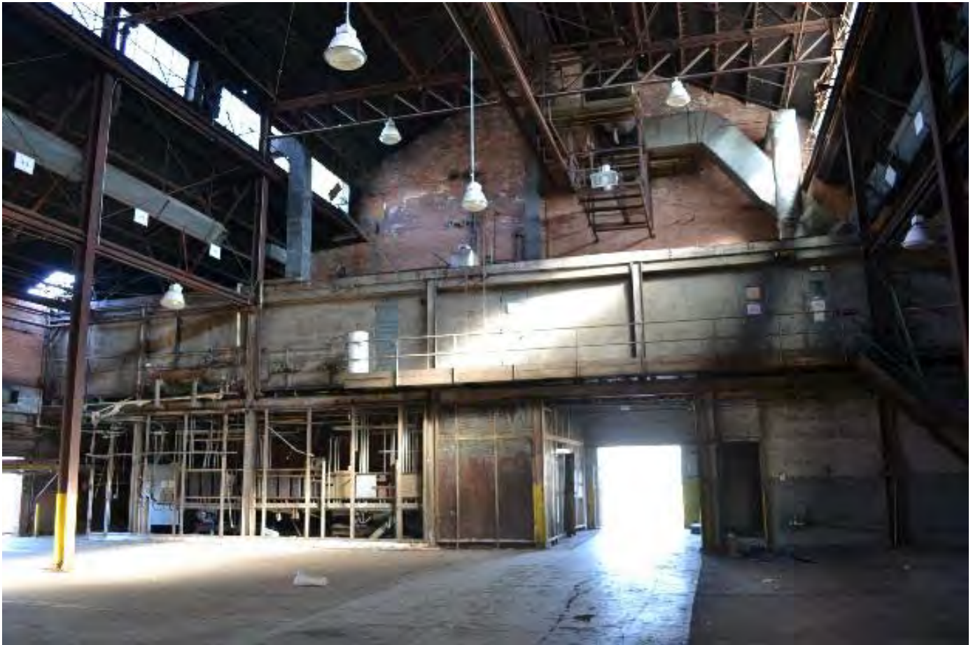
Photo 11 – 3-Bay Refined Sugar Warehouse (Resource ID 4), interior, view east
