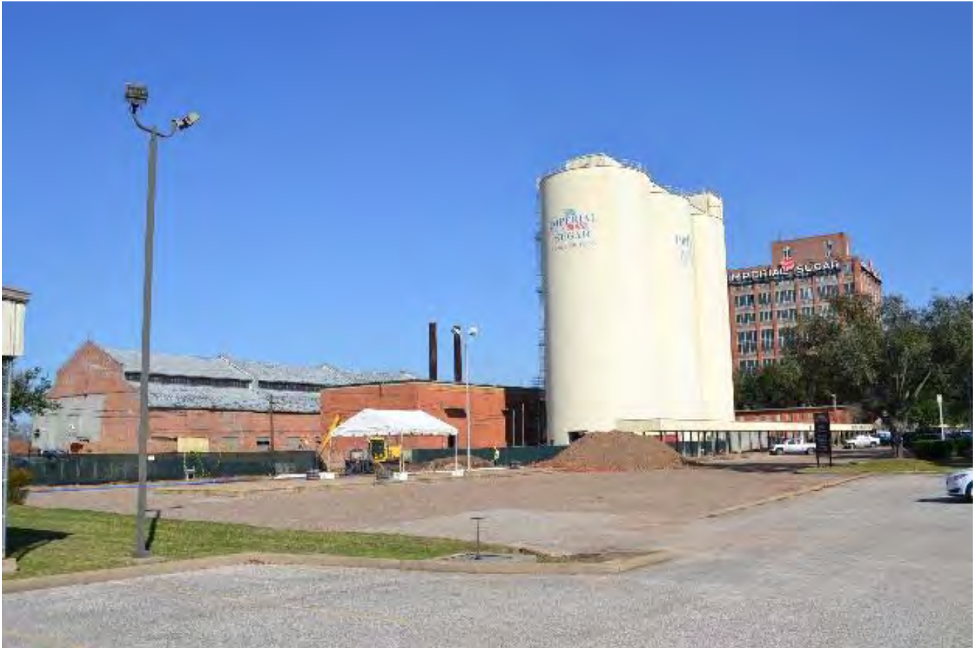
Photo 1 – Overall site, view northeast from west
