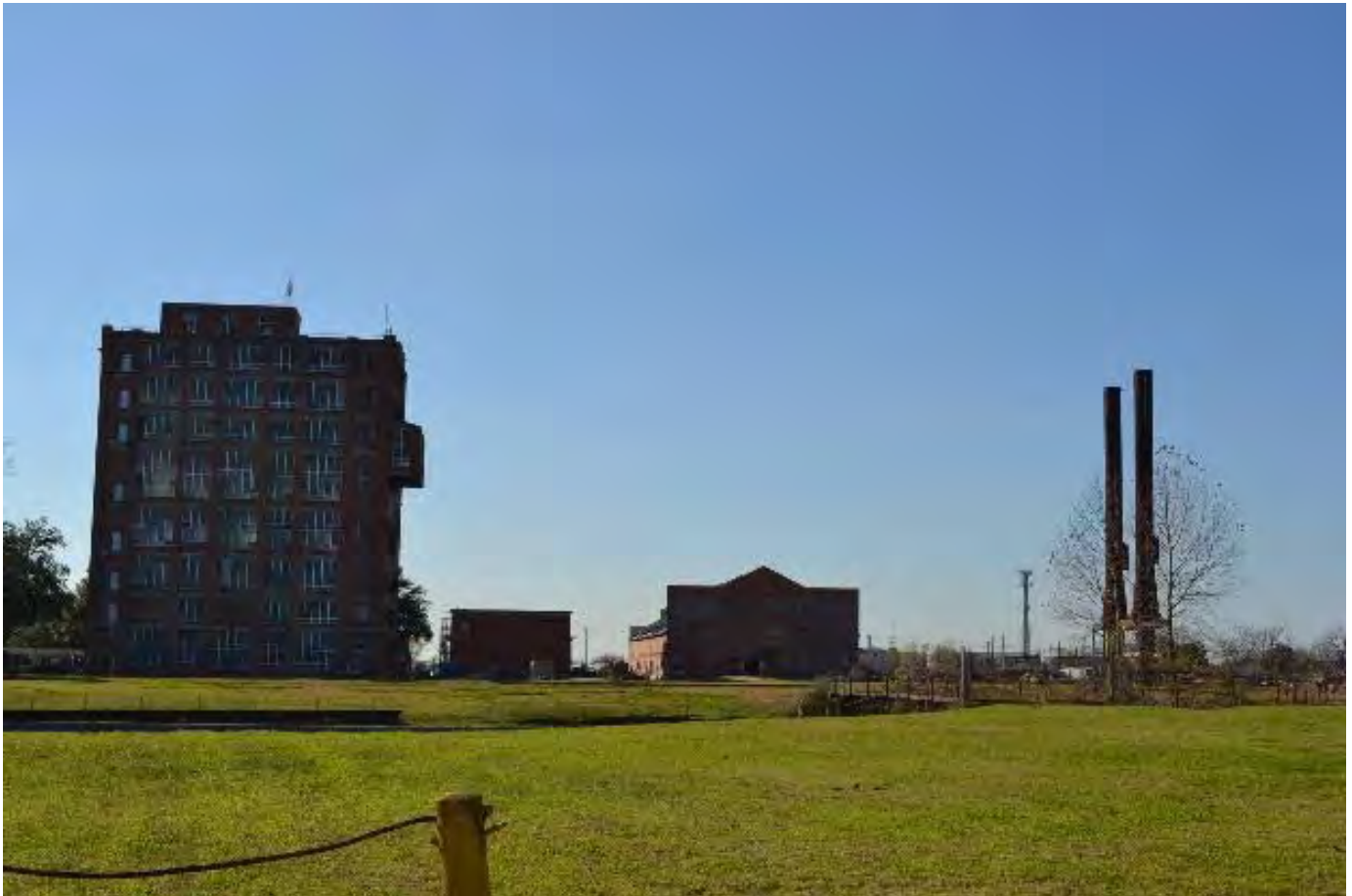
Photo 3 – Overall site, view west from east
