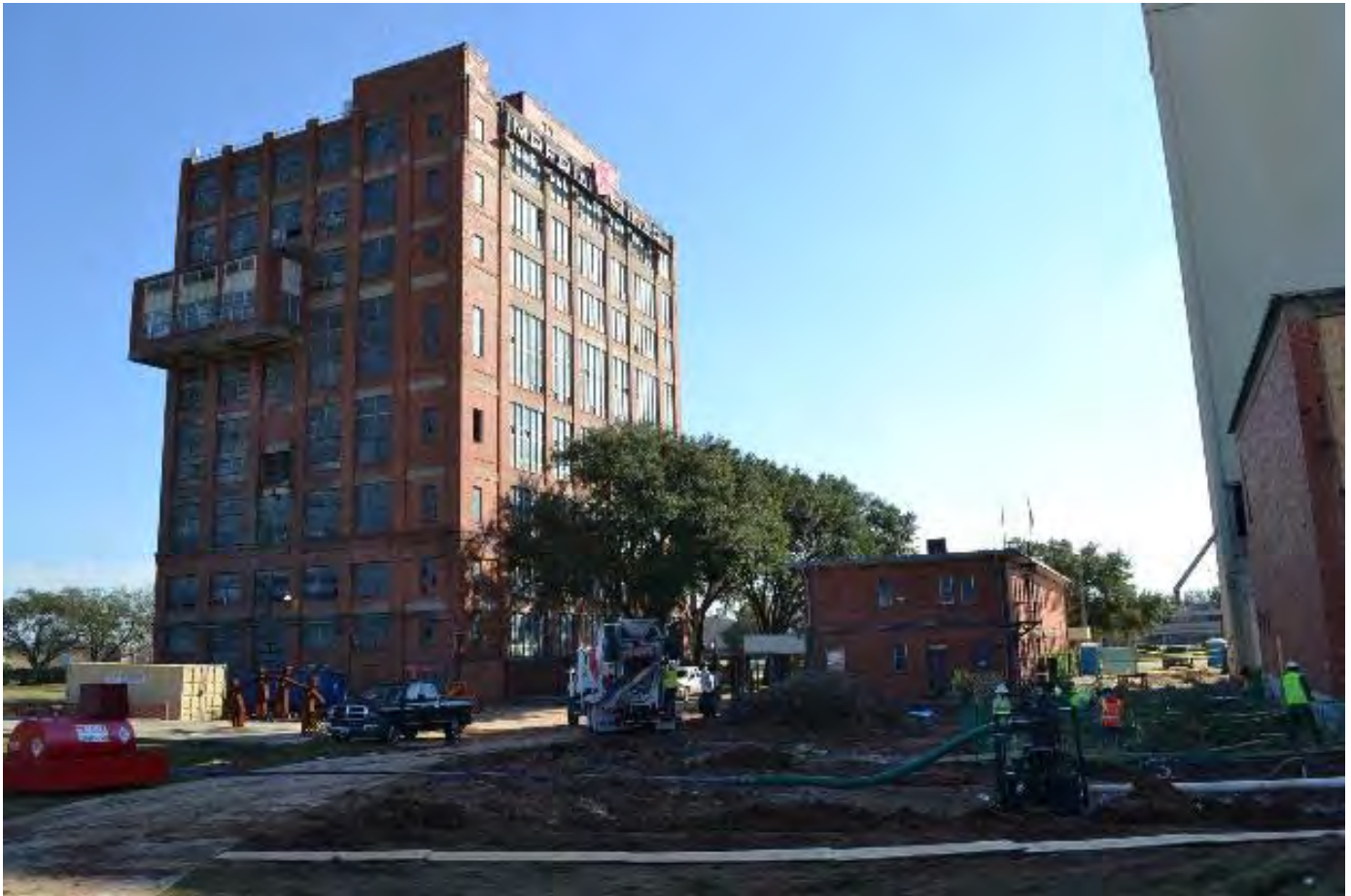
Photo 18 - Engineering Building (Resource ID 2, center), north elevation, view south
