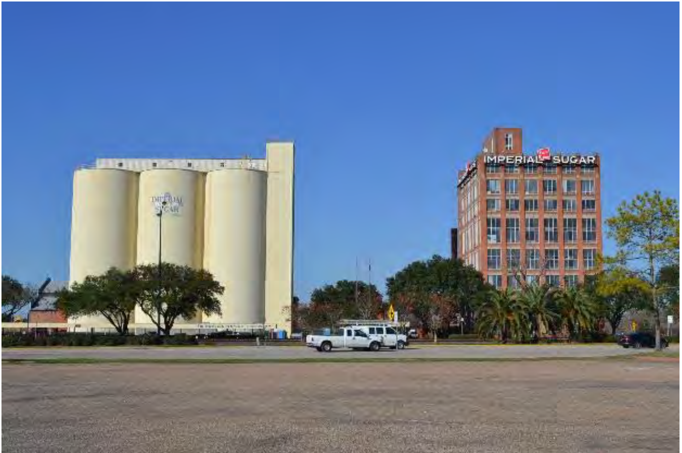
Photo 4 – Overall site, view north from south
