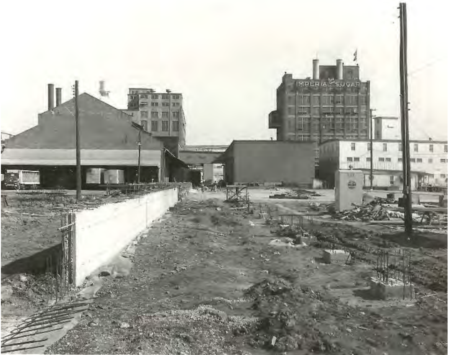
Figure 11 - During construction of a new warehouse, c. 1969. Resource ID 4 (left), Resource ID 5 (center), and Resource ID 1 (right, in background) visible. Courtesy Sugar Land Heritage Foundation.
