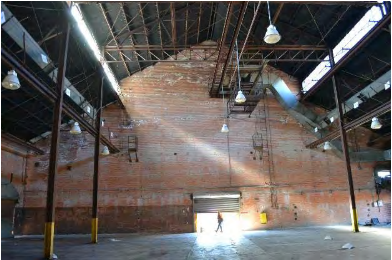
Photo 14 - 3-Bay Refined Sugar Warehouse (Resource ID 4), interior, view west
