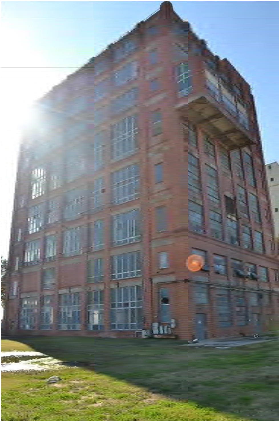
Photo 5 – Char House (Resource ID 1), east and north elevations, view southwest
