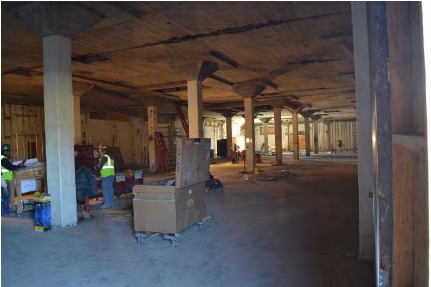
Photo 17 - Container Warehouse (Resource ID 5), interior, view west
