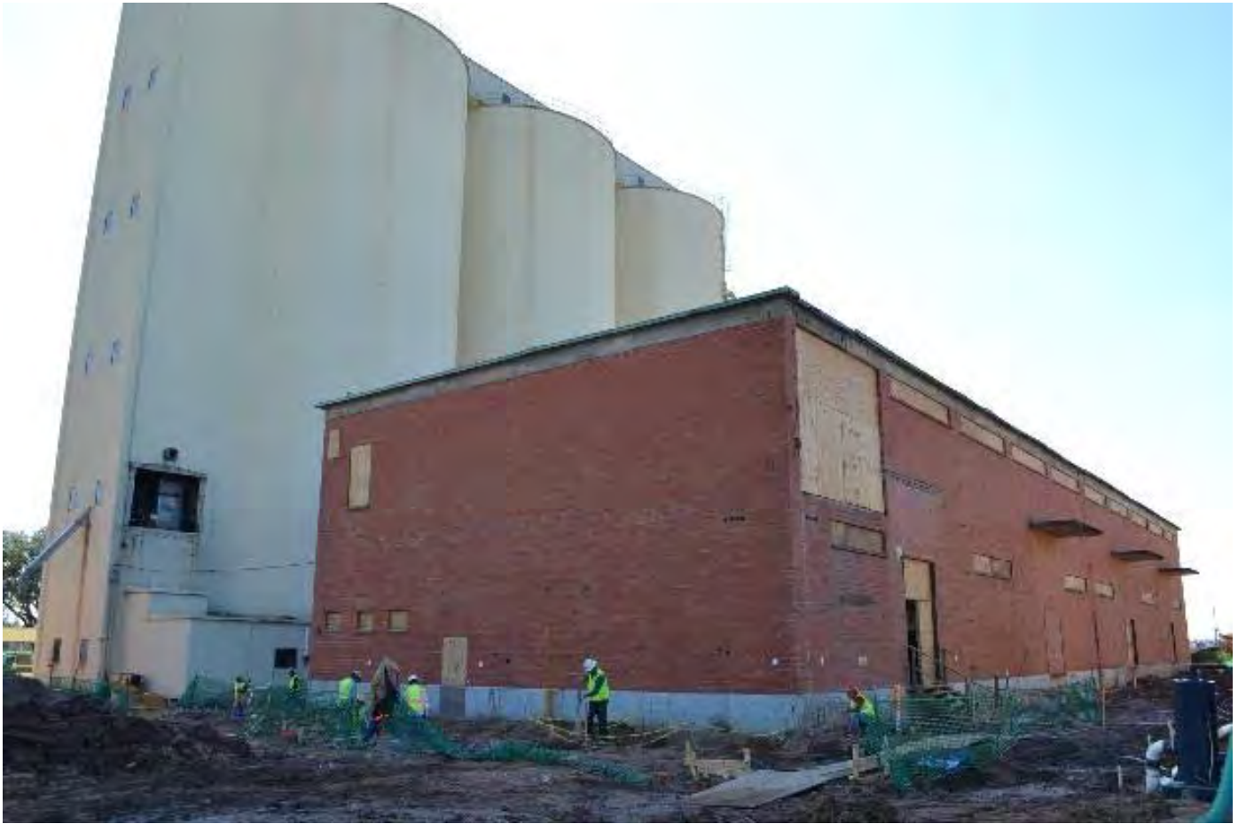
Photo 16 - Container Warehouse (Resource ID 5), east and north elevations, view southwest; silos (Resource ID 3) in background
