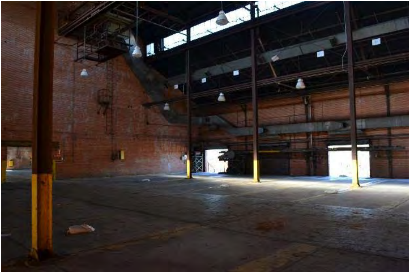
Photo 12 – 3-Bay Refined Sugar Warehouse (Resource ID 4), interior, view west
