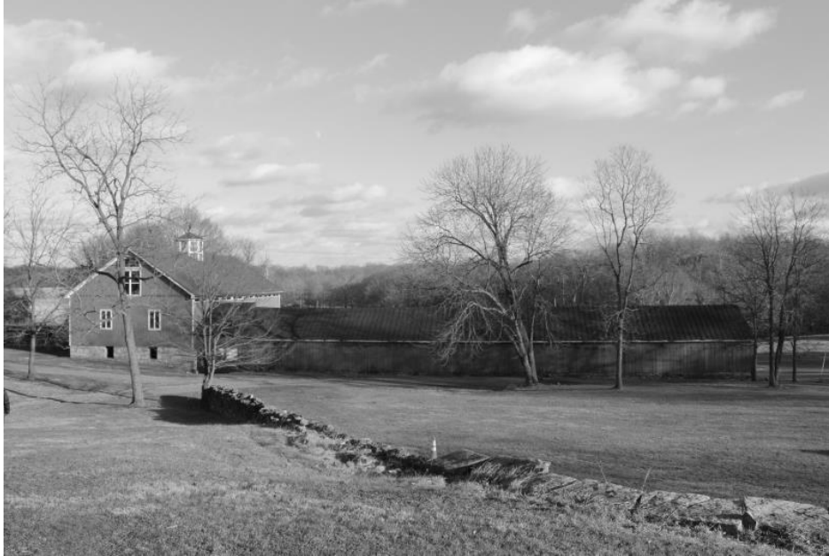
WV_Jefferson County_Wild Goose Farm_0030 Barn and attached shed, west elevation, view NE
