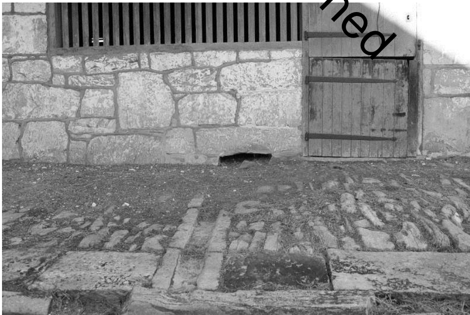
WV_Jefferson County_Wild Goose Farm_0032 Barn, south elevation forebay, detail of stone paving and drain, view N
