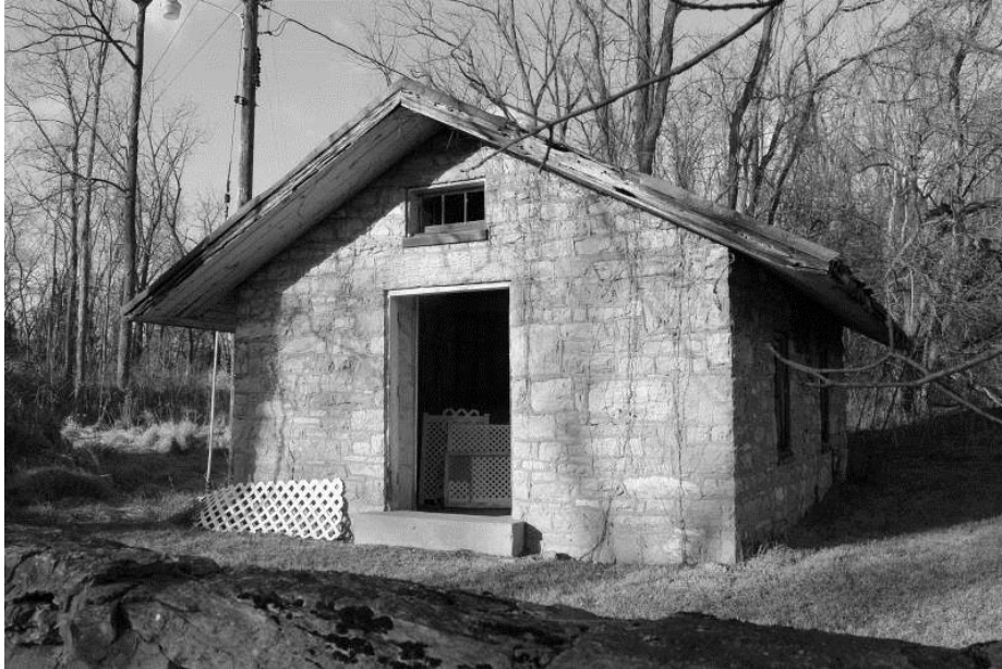
WV_Jefferson County_Wild Goose Farm_0027 Pump house, south and east elevations, view NW
