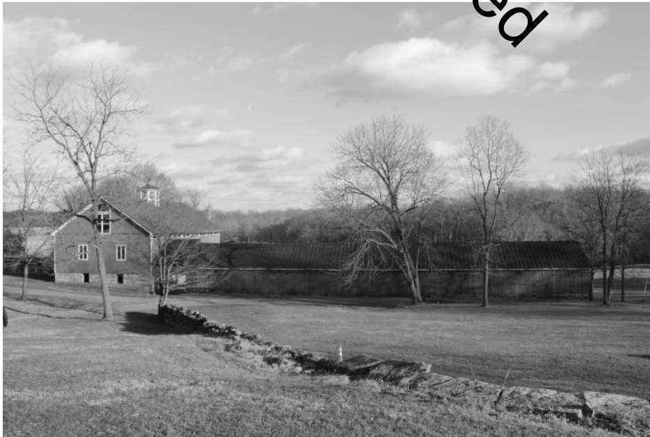
WV_Jefferson County_Wild Goose Farm_0030 Barn and attached shed, west elevation, view NE
