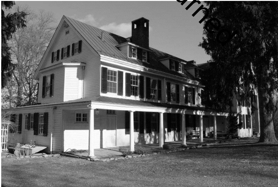
WV_Jefferson County_Wild Goose Farm_0005 Mansion exterior, west and south elevations, view NE
