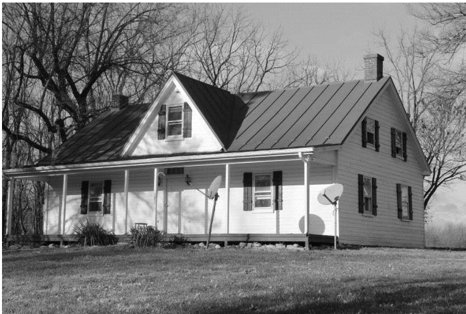
WV_Jefferson County_Wild Goose Farm_0028 Tenant house, south and east elevations, view NW
