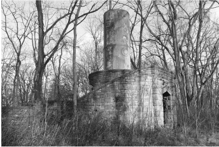
WV_Jefferson County_Wild Goose Farm_0020 Water Tower and Reservoir, view NE
