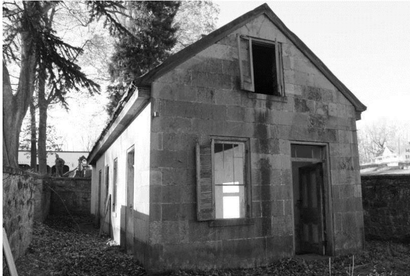
WV_Jefferson County_Wild Goose Farm_0018 Springhouse, south and east elevations, view NW
