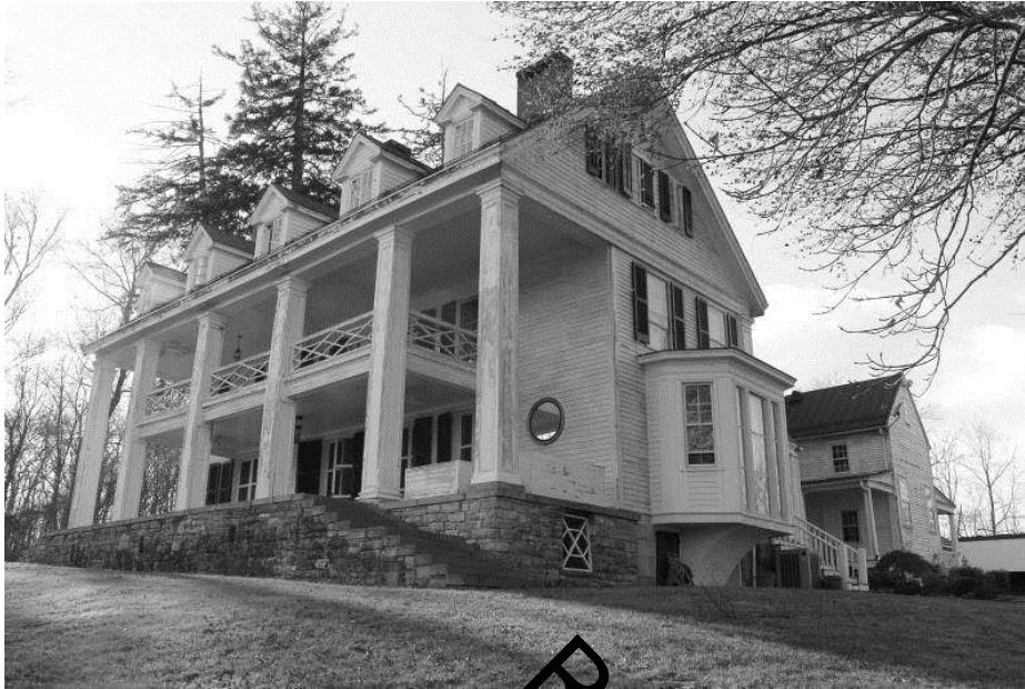
WV_Jefferson County_Wild Goose Farm_0002 Mansion exterior, east and north elevations, view SW
