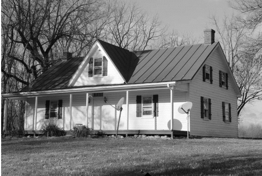
WV_Jefferson County_Wild Goose Farm_0028 Tenant house, south and east elevations, view NW
