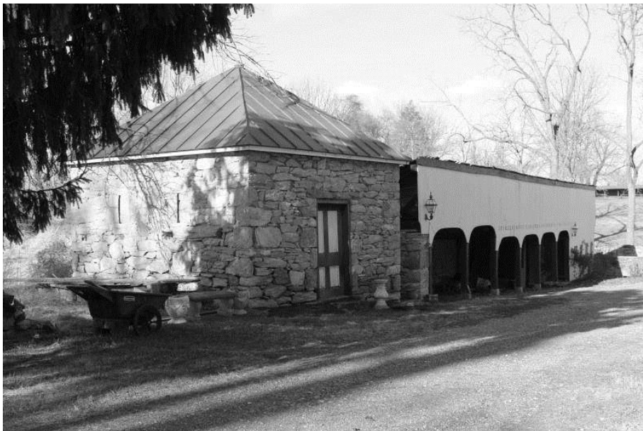
WV_Jefferson County_Wild Goose Farm_0014 Smokehouse and Carriage Shed, south and east elevations, view NW
