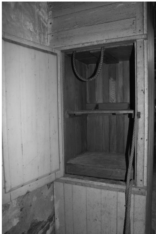
WV_Jefferson County_Wild Goose Farm_0013 Mansion interior, cellar, dumbwaiter detail, view S
