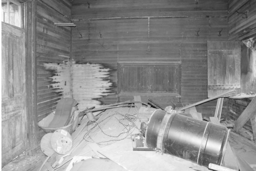
WV_Jefferson County_Wild Goose Farm_0024 Stone "plantation office," interior, view S
