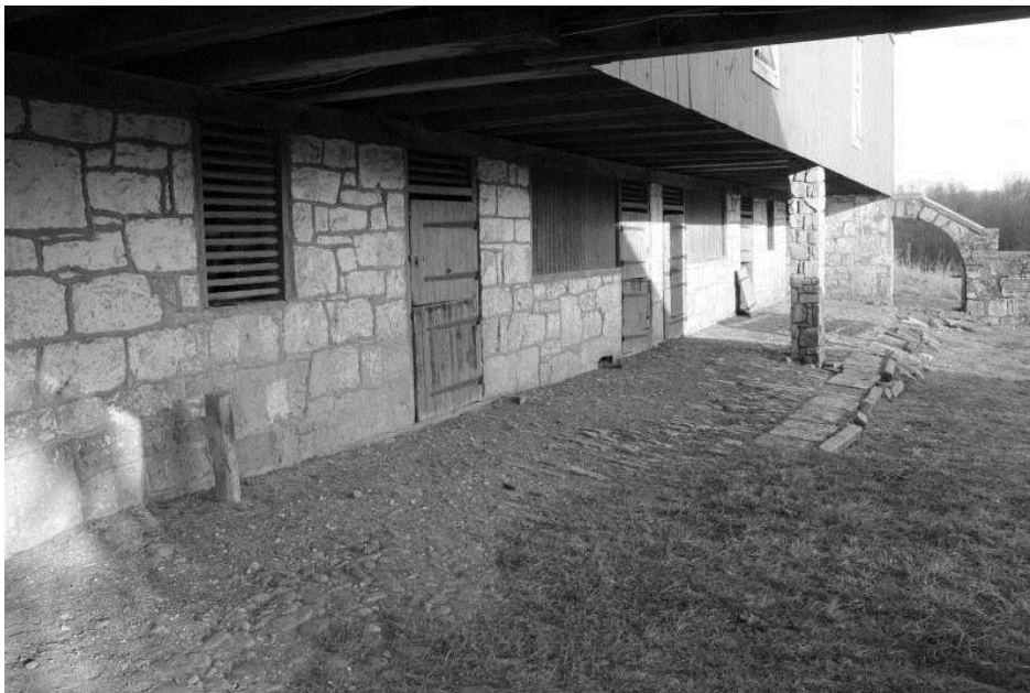
WV_Jefferson County_Wild Goose Farm_0031 Barn, south elevation forebay, view NE
