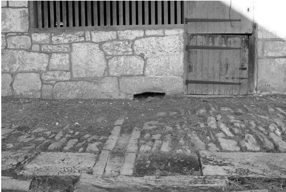
WV_Jefferson County_Wild Goose Farm_0032 Barn, south elevation forebay, detail of stone paving and drain, view N
