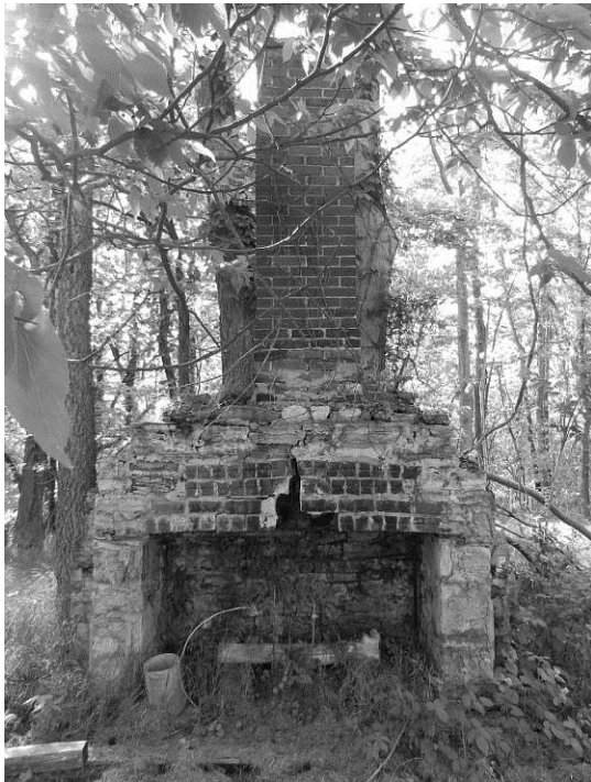
WV_Jefferson County_Wild Goose Farm_0029a Fireplace remnant; stone, brick, with iron crane
