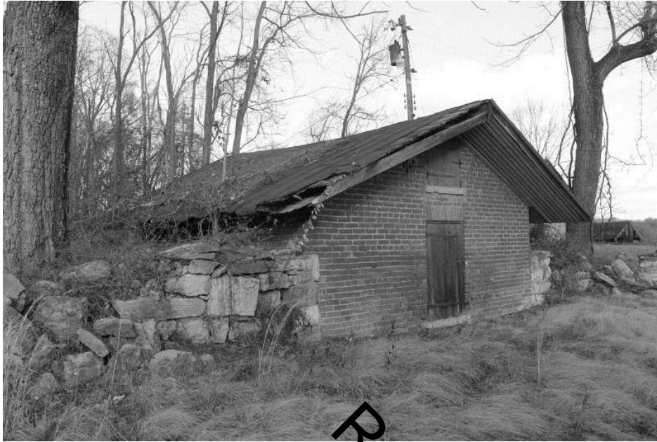
WV_Jefferson County_Wild Goose Farm_0026 Ice house, west and south elevations, view NE
