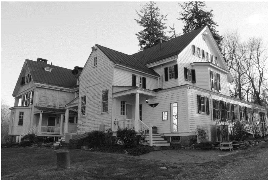
WV_Jefferson County_Wild Goose Farm_0004 Mansion exterior, north and west elevations, view SE
