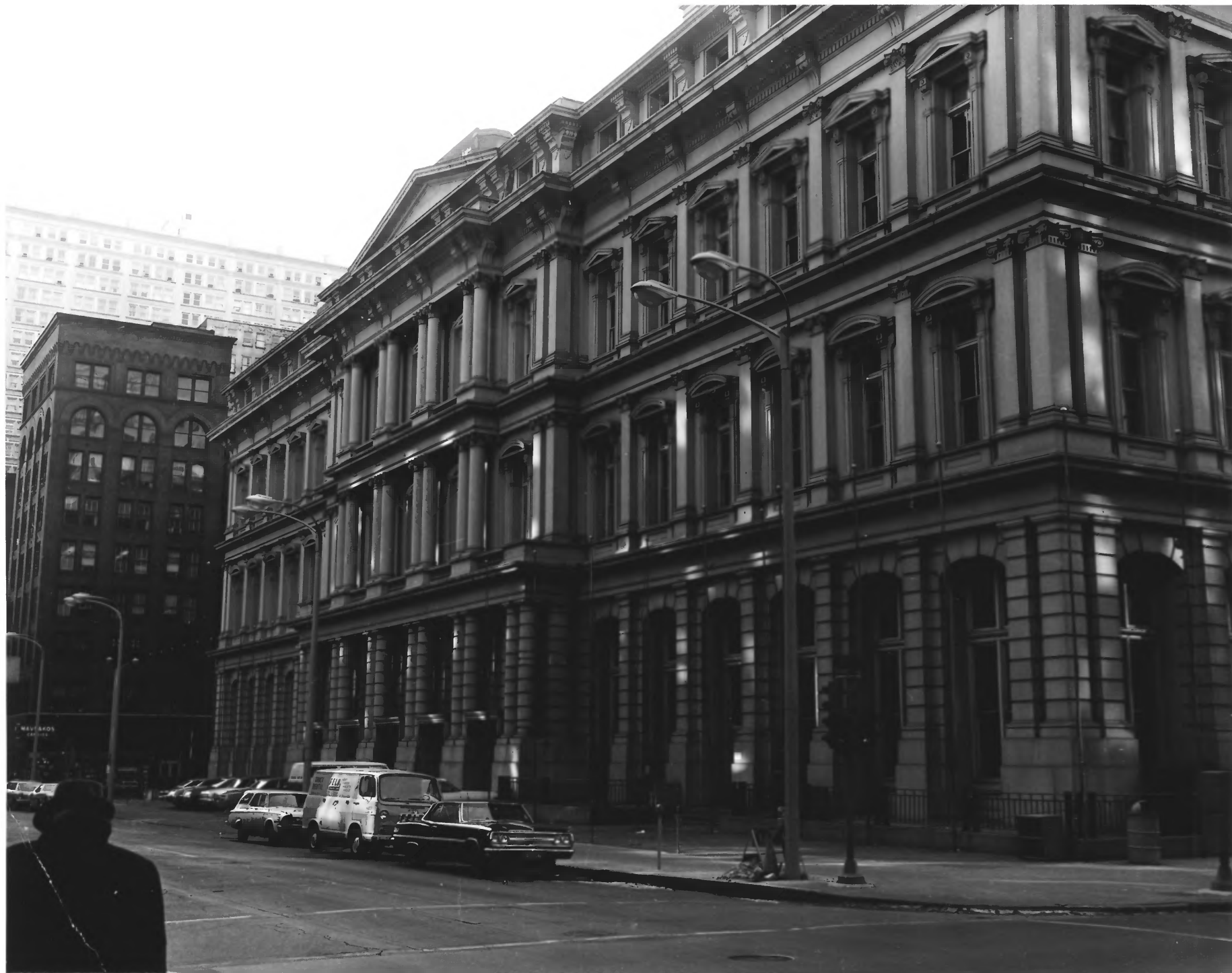
Old Post Office (Rear elevation), St. Louis, Missouri
