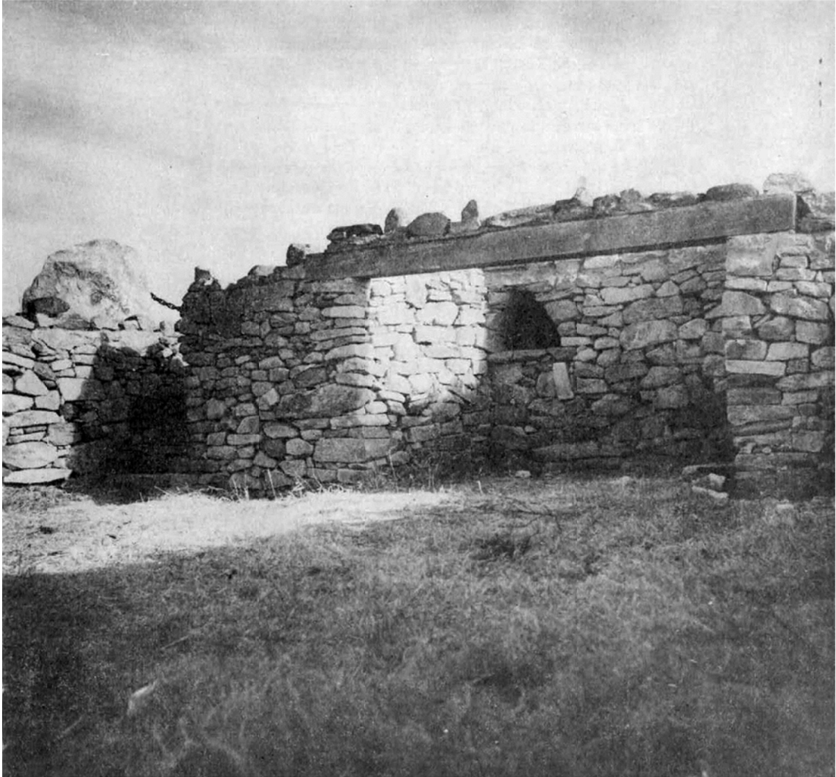
Figure 8. Photo of south wall with “beehive oven”, lintel, and commemorative boulder, view southeast from interior of North Room (source: Ricketson 1964: frontispiece).
