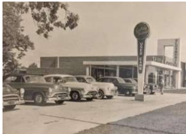
Figure 1. Griffin Motors Building, c. 1952
