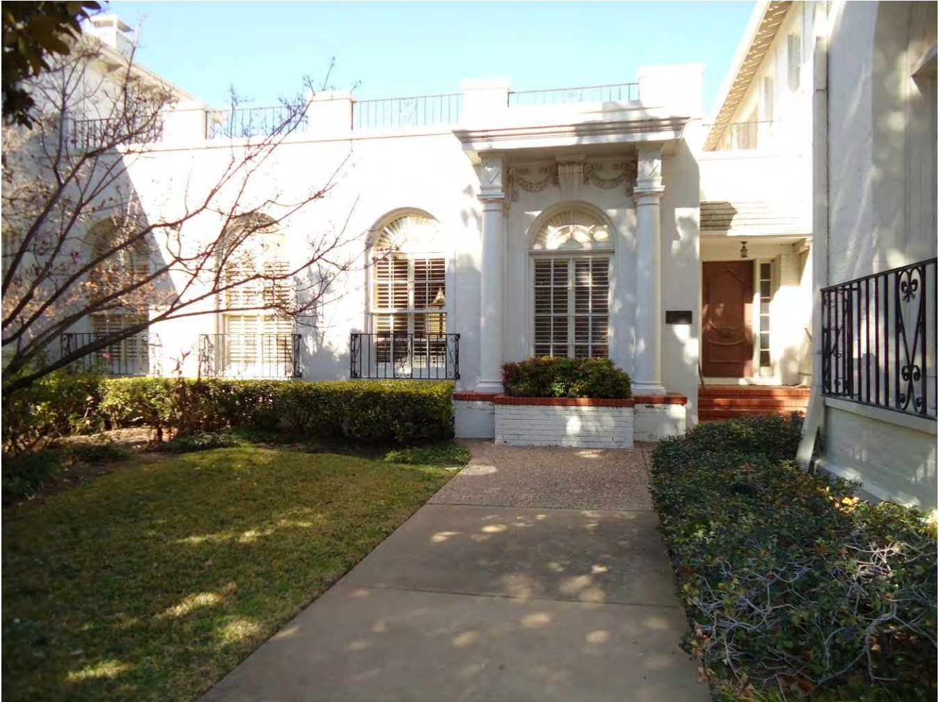
Photo 13: Bewley Hall, February 12, 2016, looking north.
