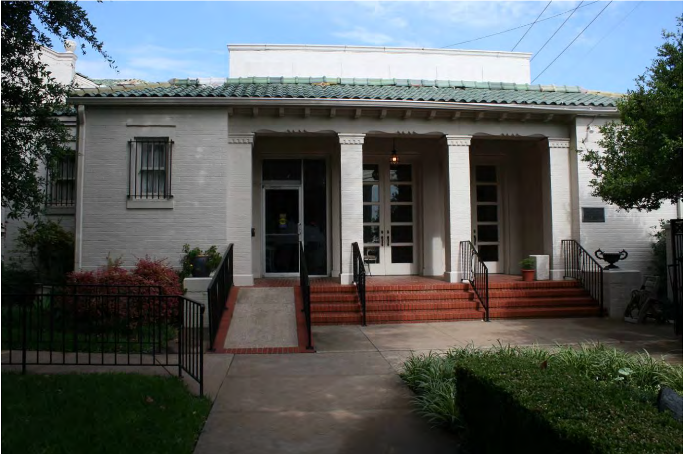
Photo 9: May R. Waples Hall and the Texas Garden, June 16, 2016, looking west.
