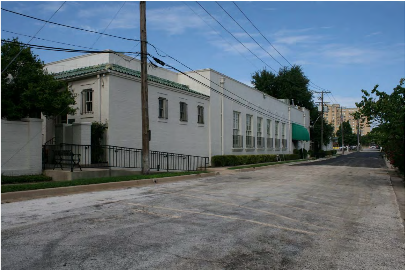
Photo 10: May R. Waples Hall (north elevation) and Woman's Club Drive (formerly Tucker Street), June 16, 2016, looking southwest.
