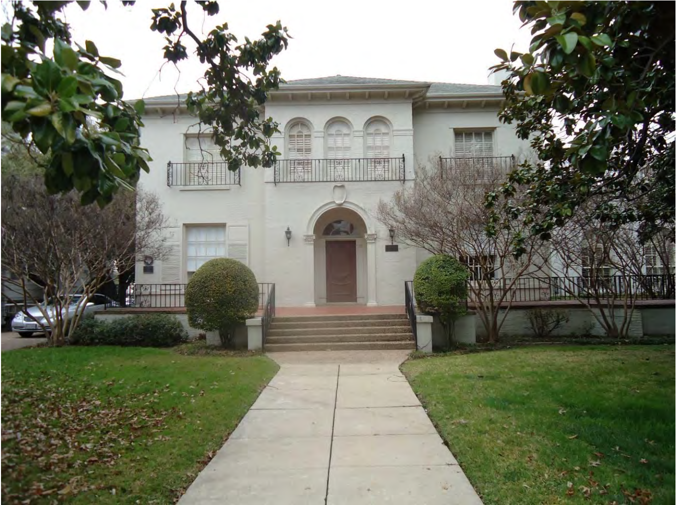
Photo 17: Ida Saunders Hall, March 18, 2015, looking north.
