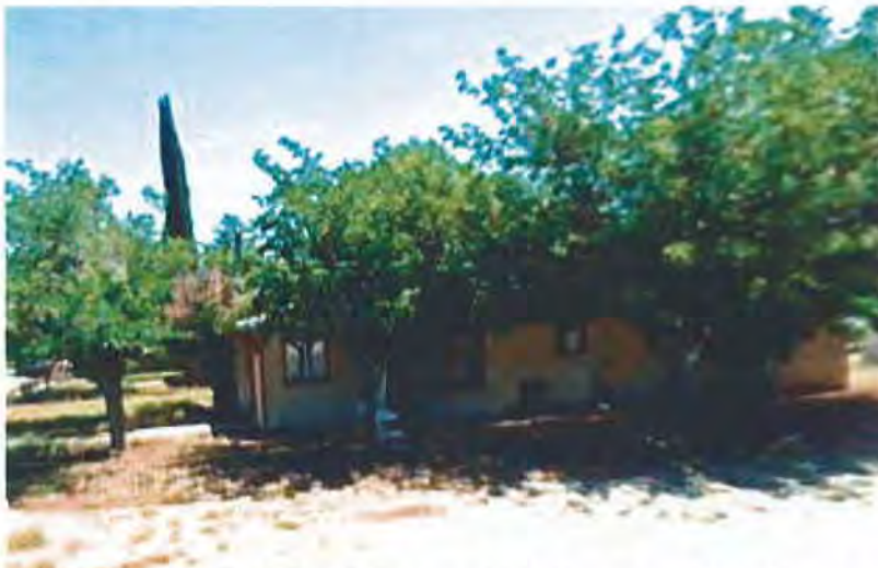
Figure 1. House at 1515 Main St. in 2008 showing enclosed front porch. Source: Google, 2008)
