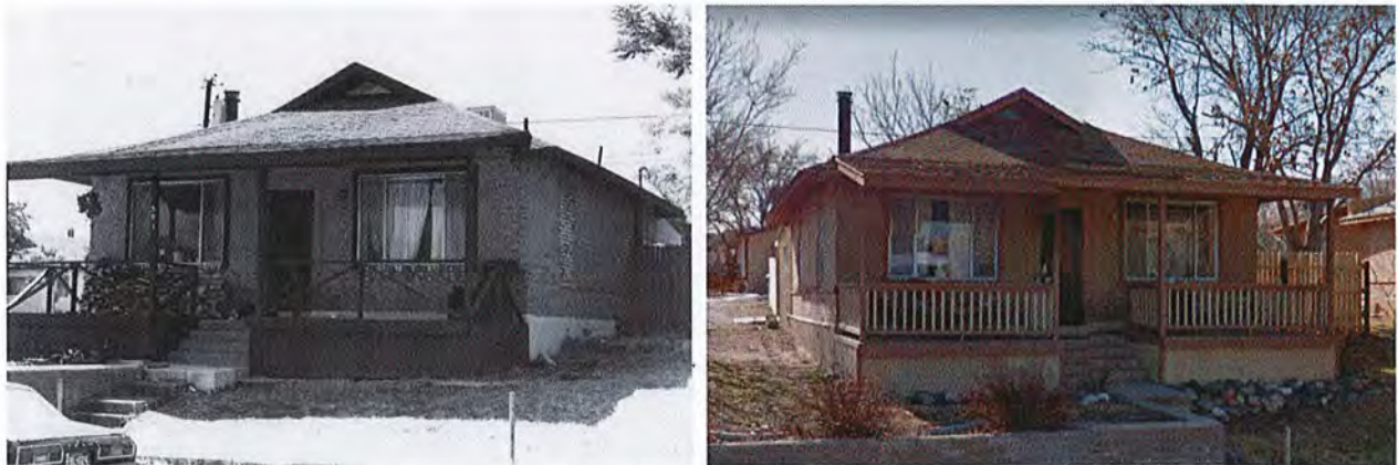
The house at 501 1st North Street from the 1989 historic building survey of Clarkdale (left) and as it appears in 2019 (right).
