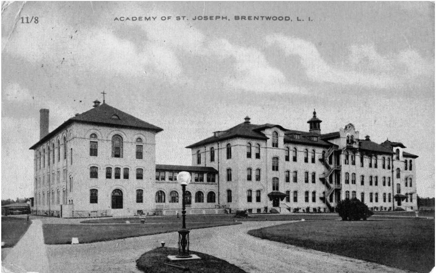
Figure 1. Exterior, Rear view of Assembly Hall and Elementary School, c 1903-12, facing NW.
