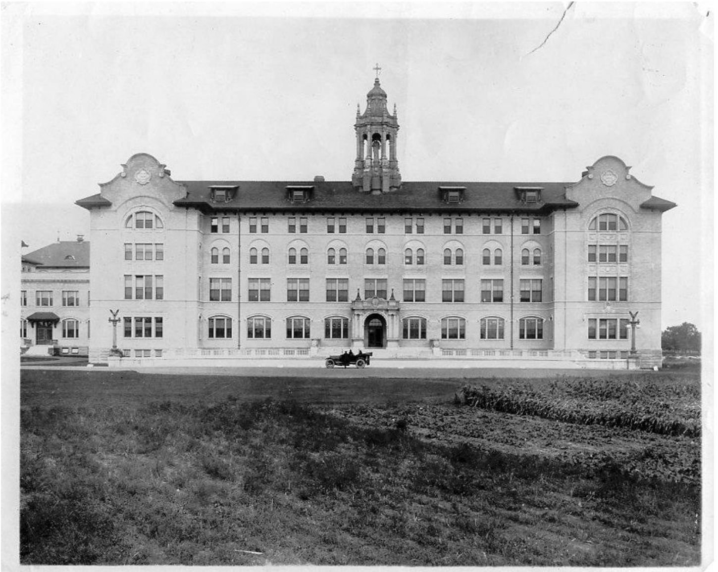
Figure 3. Exterior, Academy High School main building, c 1913, facing SW.
