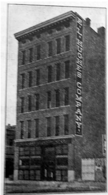
Figure 4. E. L. Hughes Co. (CD 1907: 2146) South Facade
