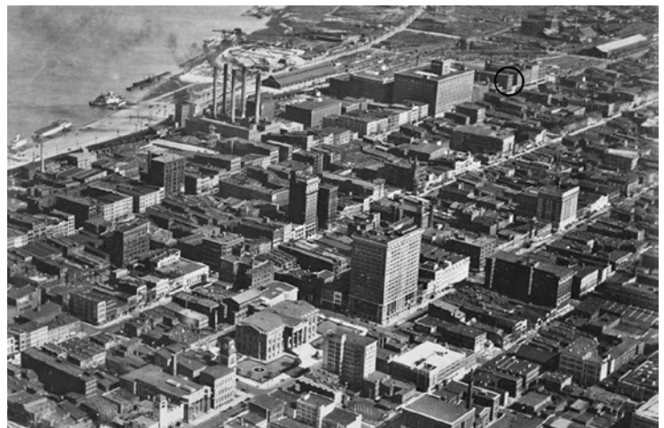
Figure 3. Louisville, Kentucky aerial photograph circa late 1930s (circle locates the E. L Hughes Building)
