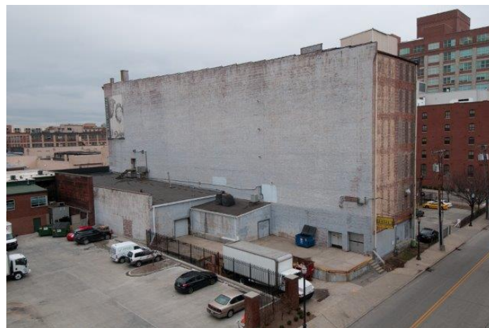
Rear and east side, view to southwest (photo 10)
