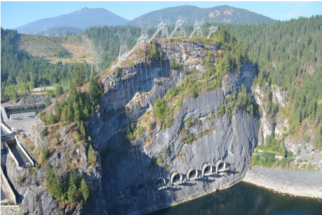
Photo 8 of 25: (WA_PendOreille_BoundaryDam__008) Boundary Dam, Powerhouse formation (Left Abutment), showing Transformer Bays, Transmission Line, camera facing West, from Vista House Overlook (A)
