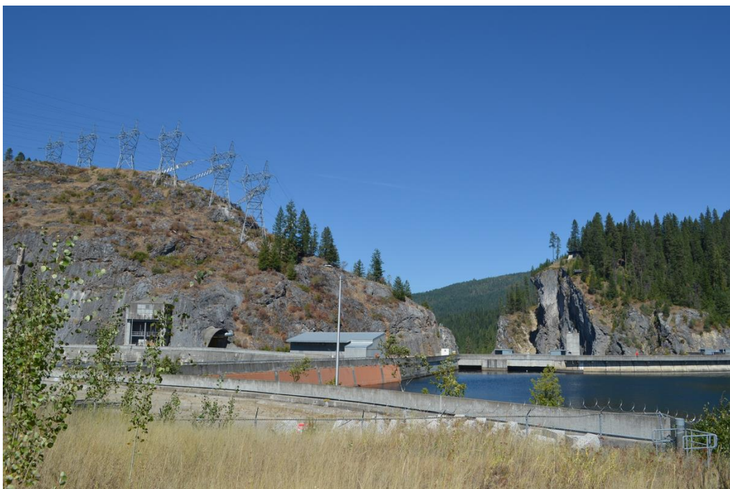
Photo 3 of 25: (WA_PendOreille_BoundaryDam__003) Boundary Dam, Forebay, Towers, camera facing NW, from Forebay Area (A)
