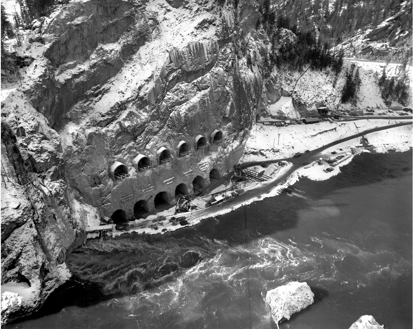
FIGURE 14. Historic Photo, Transformer Bays, Draft Tubes, and Tailrace Construction, February 20, 1967 (Seattle Municipal Archives, Image No. 185539)
