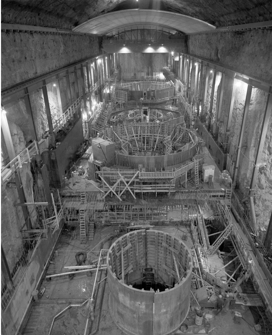
FIGURE 11. Historic Photo, Machine Hall Construction August 1, 1966, Unit 51 in Foreground (Seattle Municipal Archives, Image No. 184611)
