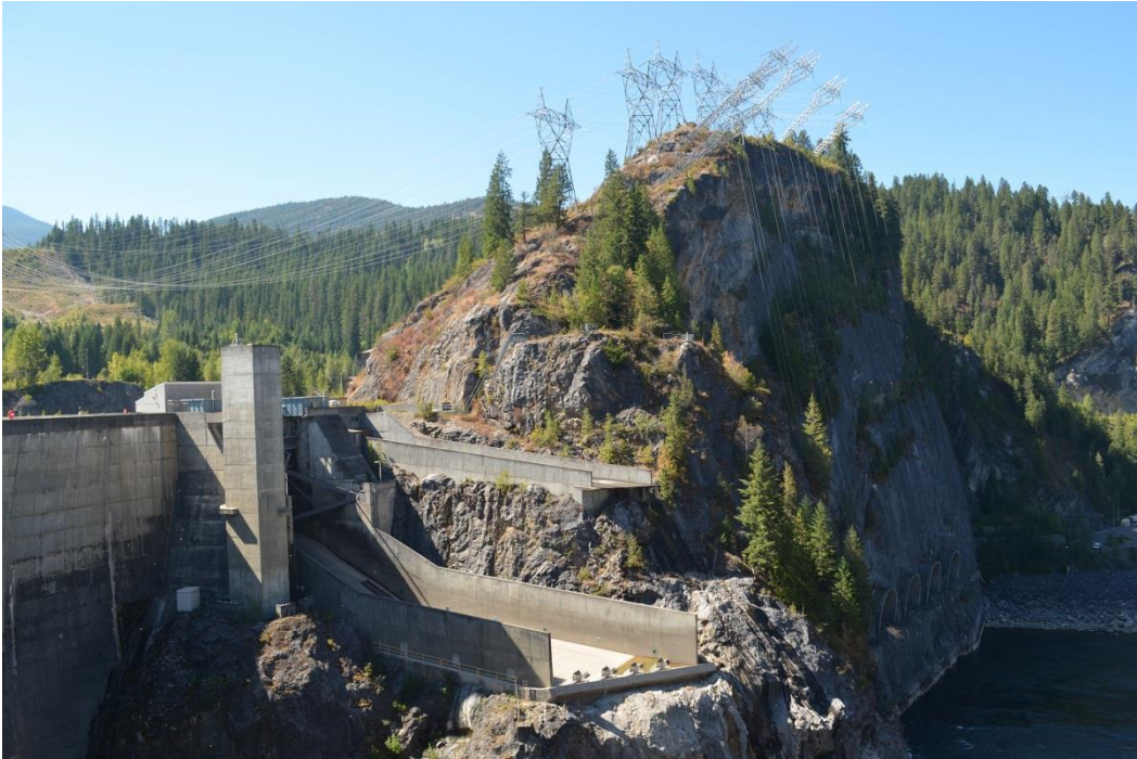
Photo 7 of 25: (WA_PendOreille_BoundaryDam__007) Boundary Dam, Elevator Tower, Left Spillway, Skimmer Gate, Transmission Line, Powerhouse formation, camera-looking West, from Vista House Overlook (A)
