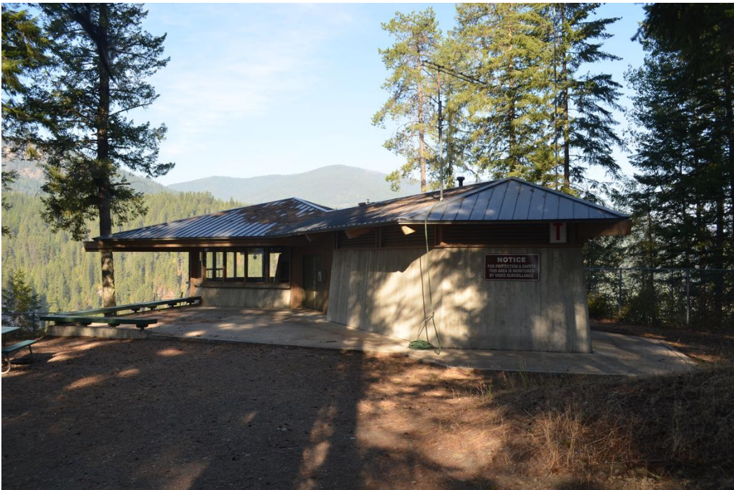
Photo 19 of 25: (WA_PendOreille_BoundaryDam__019) Vista House, camera looking N from trailhead (A)
