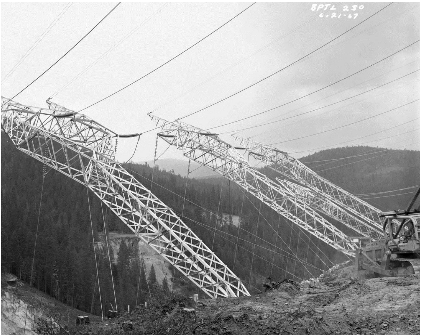
FIGURE 27. Historic Photo, Boundary Dam Transmission Line, "Picklefork" Cantilevered Towers, Looking SE, June 21, 1967 (Seattle Municipal Archives, Image No. 182751)
