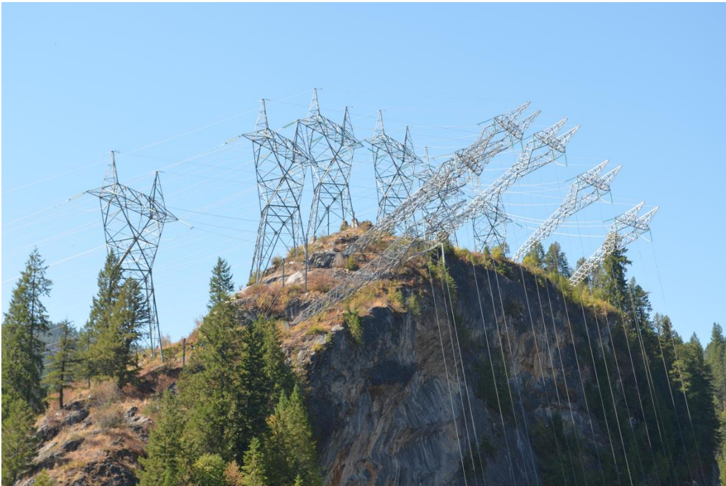
Photo 23 of 25: (WA_PendOreille_BoundaryDam__023) Boundary Dam Transmission Line, Pickleforks, camera looking NW from dam crest (A)
