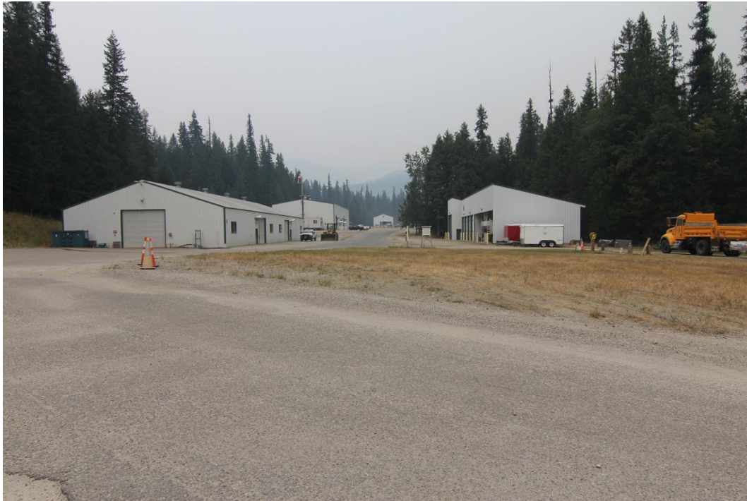
Photo 25 of 25: (WA_PendOreille_BoundaryDam__025) Boundary Dam Operations and Maintenance Service Area, General View, camera looking N from Access Road (K)
