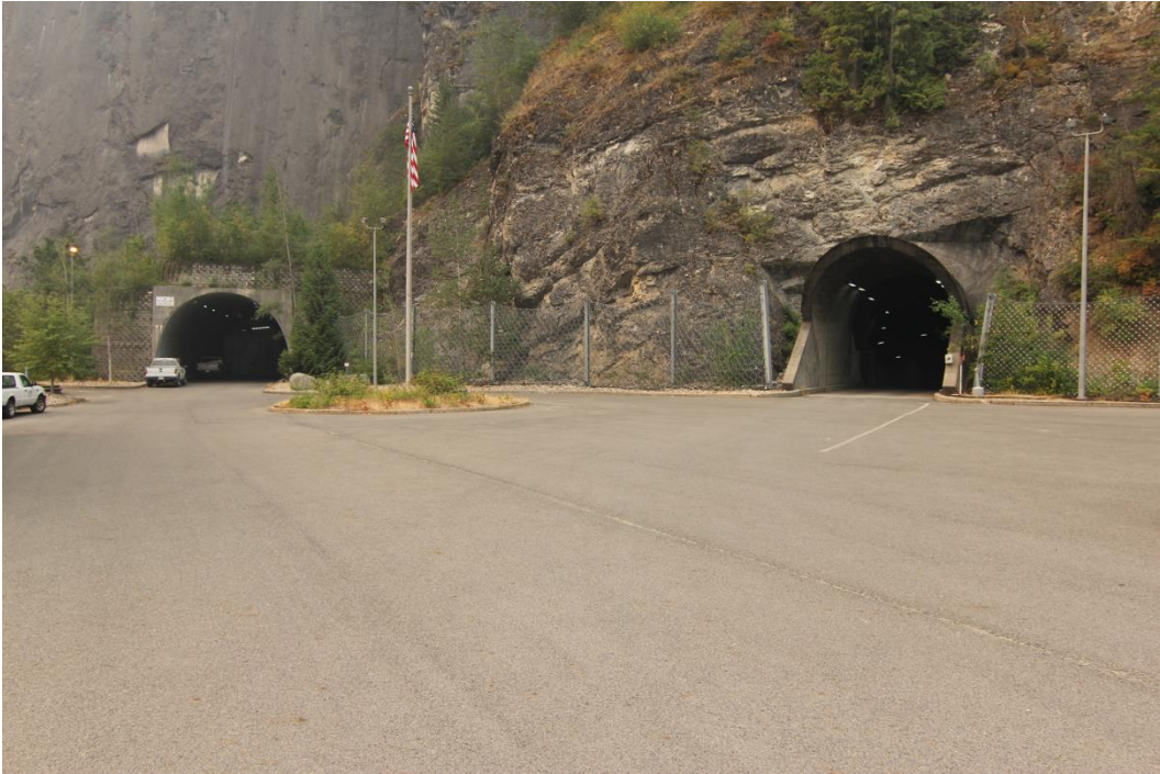
Photo 11 of 25: (WA_PendOreille_BoundaryDam_011) Boundary Dam, Powerhouse Access Tunnels with "Bonnets," camera looking SW from Tailrace Recreation Area/Access Road (K)
