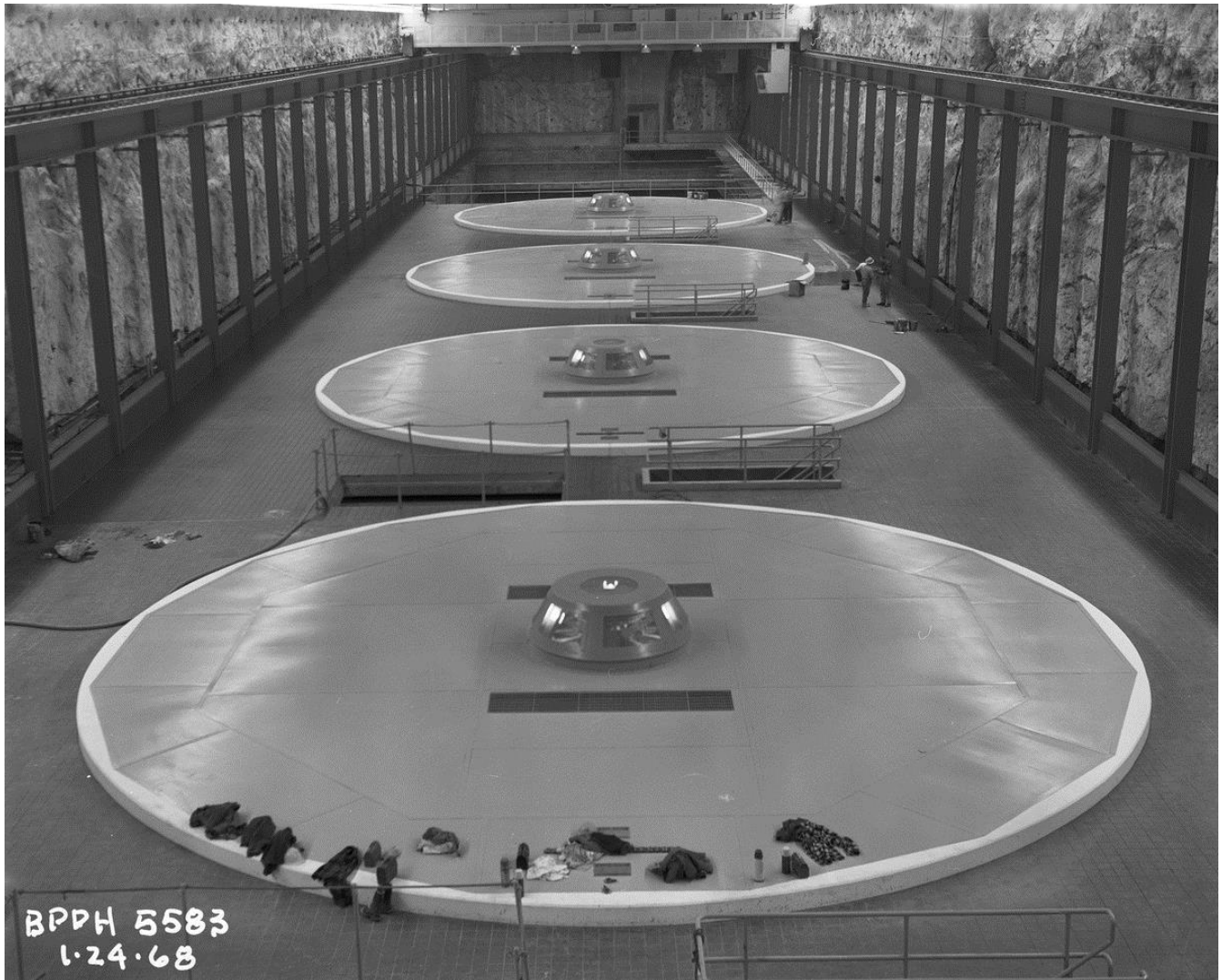
FIGURE 13. Historic Photo, Machine Hall Construction January 24, 1968, showing Units 51-54, with cavity for later expansion in distance (Seattle Municipal Archives, Image No. 183480)
