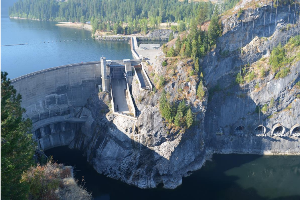
Photo 5 of 25: (WA_PendOreille_BoundaryDam__005) Boundary Dam, Reservoir, Forebay, Transformer Bays (Powerhouse), overview, camera facing SW, from Vista House Overlook (A)
