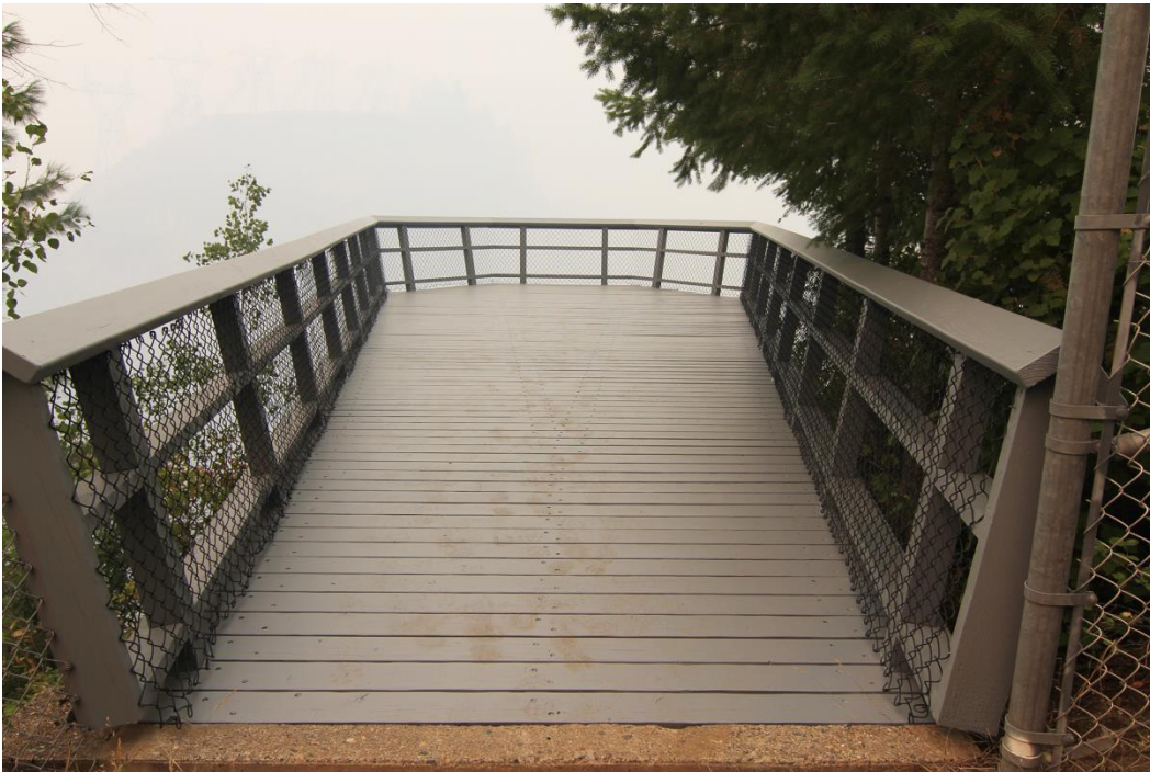
Photo 21 of 25: (WA_PendOreille_BoundaryDam__021) Vista House Overlook platform, camera looking W (K)
