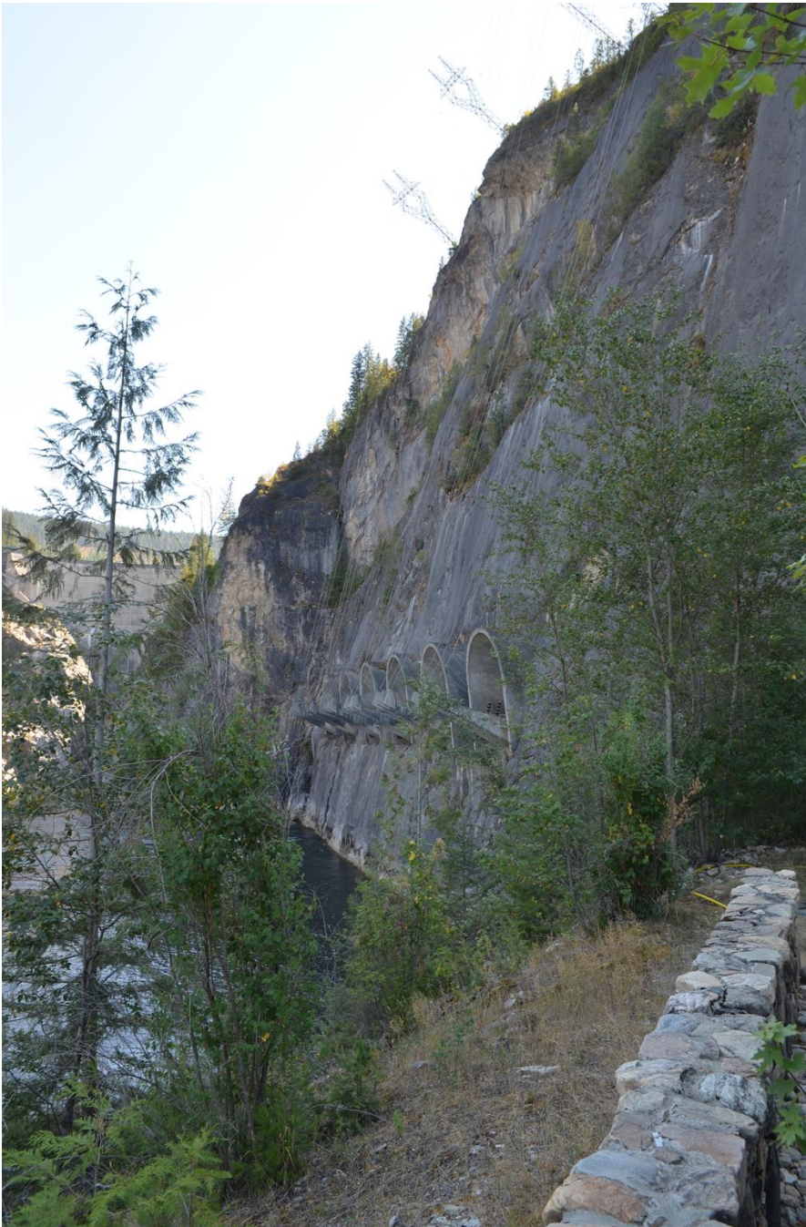
Photo 4 of 25: (WA_PendOreille_BoundaryDam_004) Boundary Powerhouse, Transformer Bays (Bonnets) and Picklefork Towers, camera facing SE from Tailrace (A)
