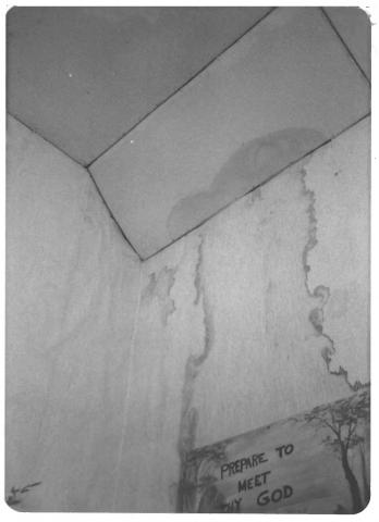
10-27-80 Interior of shurch showing stains on Wall + ceiling from rains in early 1980. a hen Cedar roof was installed in Sept 1980
