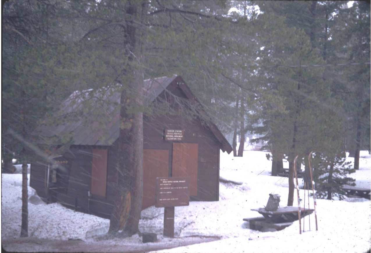
Figure 4. Southeast corner, showing the corrugated iron roof and exposed rafter ends, camera facing northwest, 1972. Photographer: Wymond Eckhart. Devils Postpile National Monument, Wymond Eckhart slide collection.
