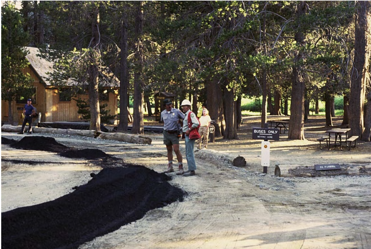
Figure 5. Northwest corner during the 1979 renovation, showing the new roof, siding, fascia, windows, door, and raised foundation, camera facing southwest. Photographer: Wymond Eckhart. Devils Postpile National Monument, Wymond Eckhart slide collection.
