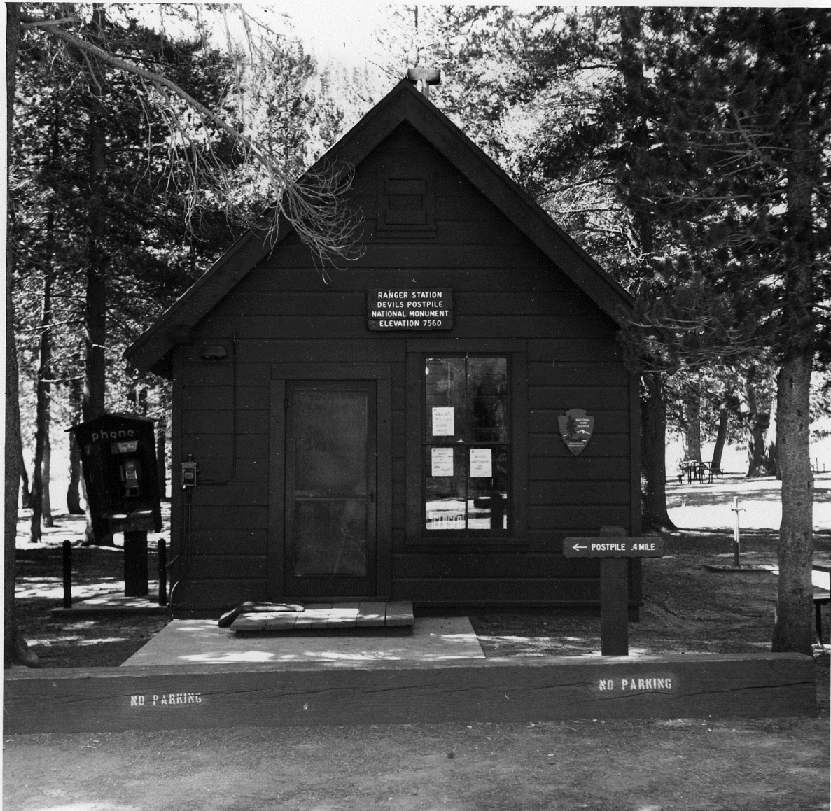
Figure 3. East elevation (front), showing the original siding, door and window configuration, and wood slat air vent, camera facing west, 1976. Photographer unknown. Scanned from archived image, Sequoia and Kings Canyon National Parks Archive.
