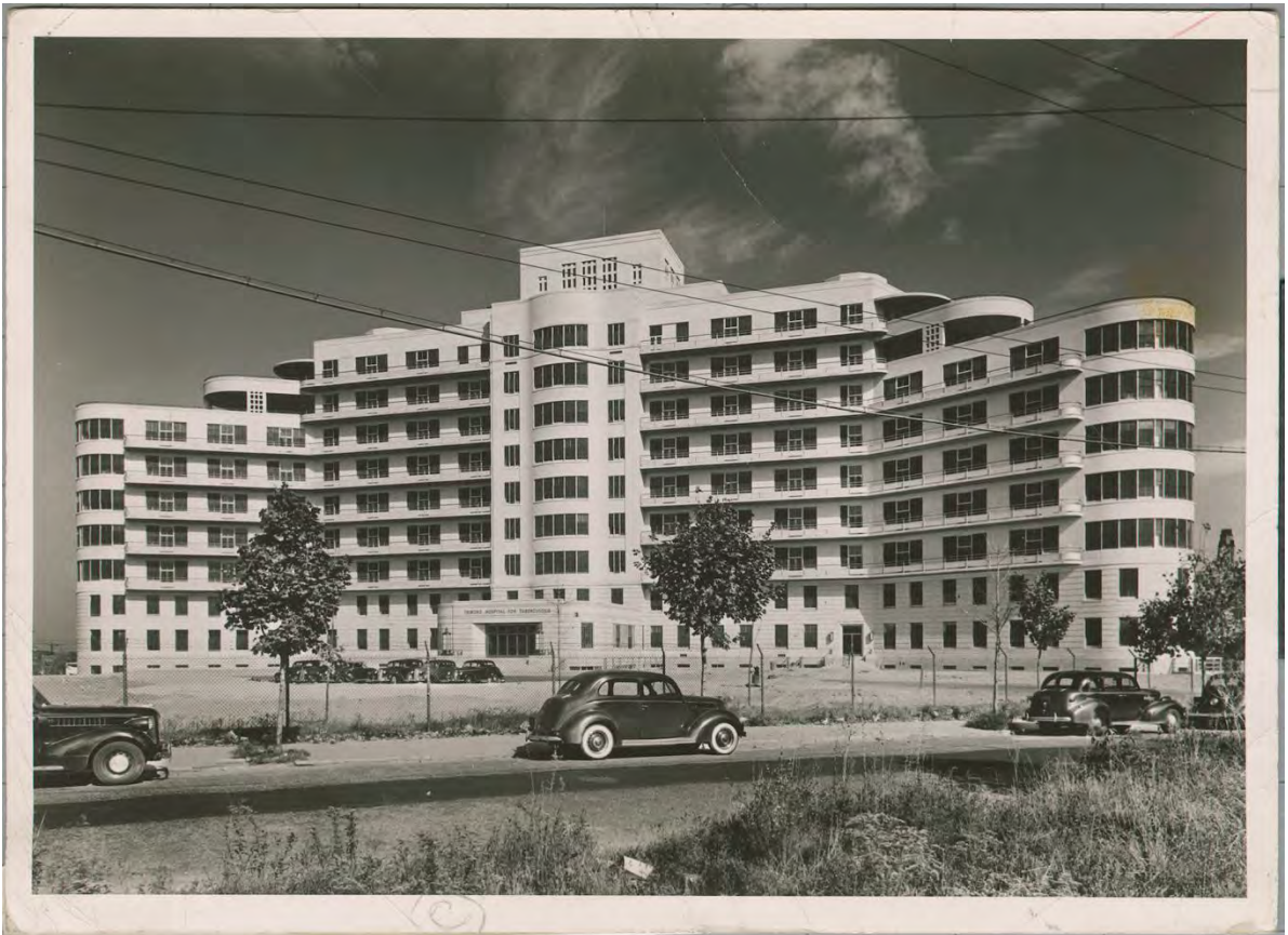
H8. The Triboro Hospital for Tuberculosis, photographed as it neared completion in the fall of 1940. Using this photo, the Department of Public Works submitted the hospital to the Annual Building Awards of the QueensBorough magazine (December 1940) p. 29, for which the building won a bronze plaque. Collection: Department of Public Works, Municipal Archives.
