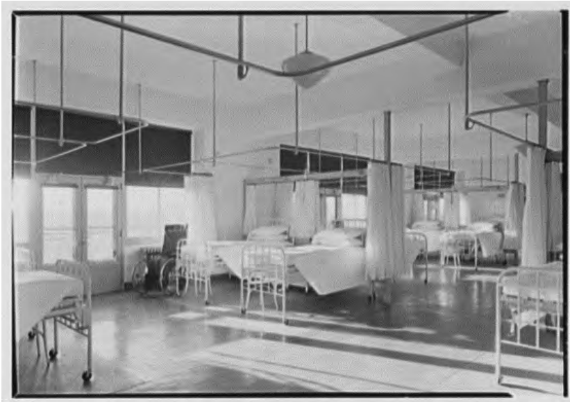
H10. 24-bed ward. The Triboro Hospital was thoroughly documented by the architectural photographers Gottscho-Schleisner on behalf of Eggers and Higgins. Many of the images were reproduced in a feature article in The Architectural Forum , February 1941. Gottscho-Schleisner Collection, Library of Congress.
