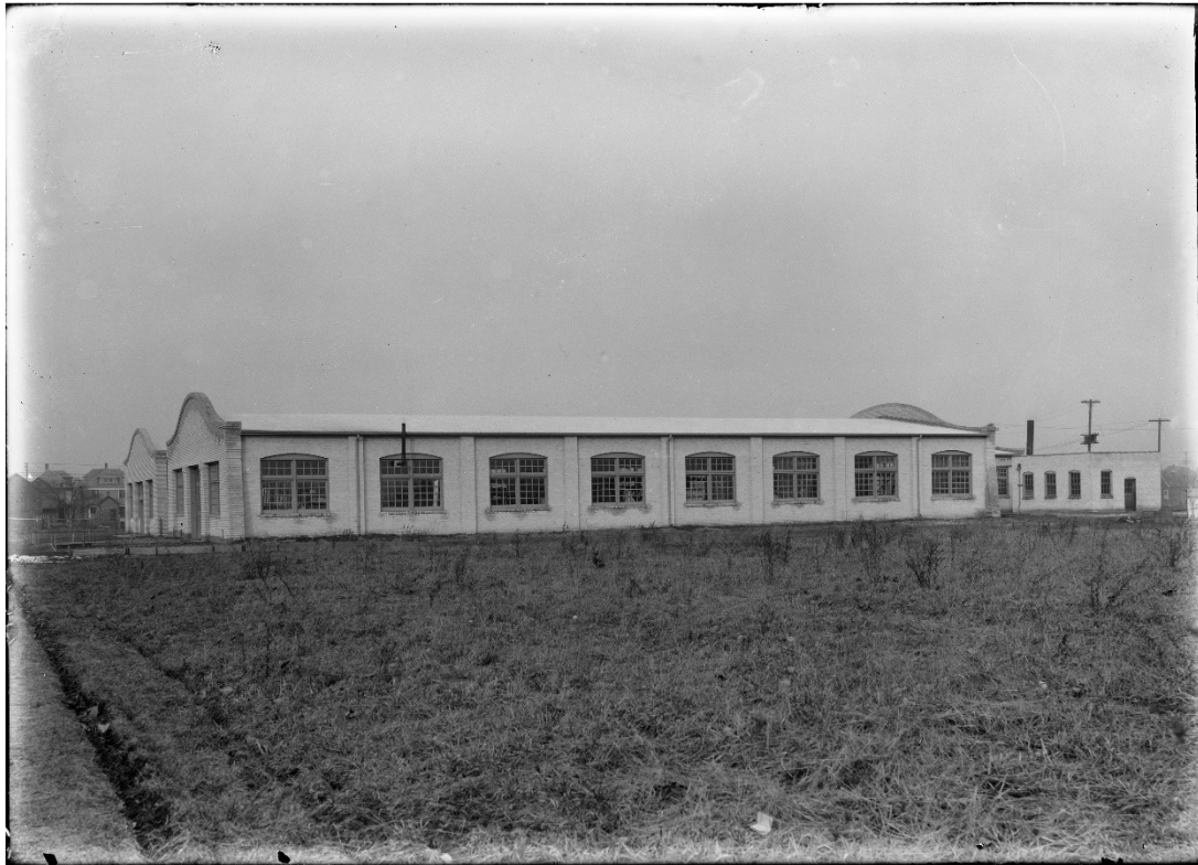
Figure 2: Wright Company Factory, 1911, after Building 2 addition was completed, showing the south side façade and the small power house located to its rear, east side.
