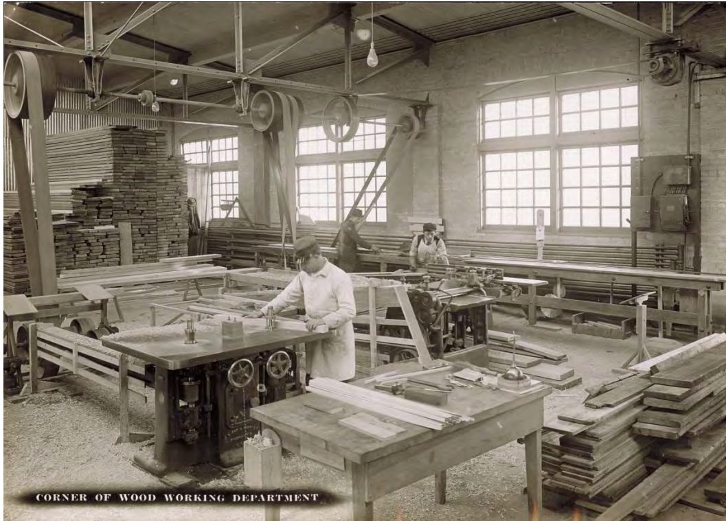
Figure 5: Wright Company Factory, view of the Woodworking Department after the completion of Building 2 addition.
