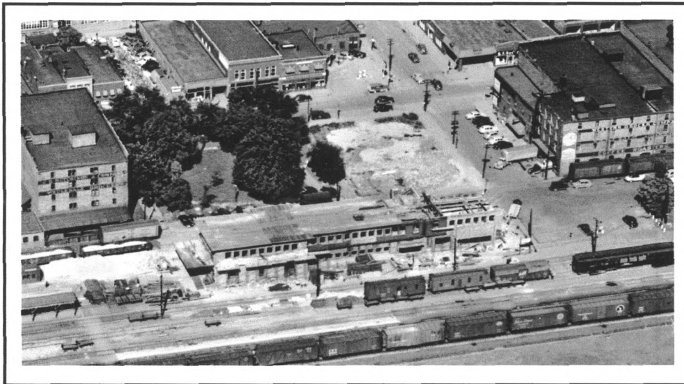
Old Depot during partial demolition in May 1950 (Courtesy of Michael W. Lemberger Private Collection)
