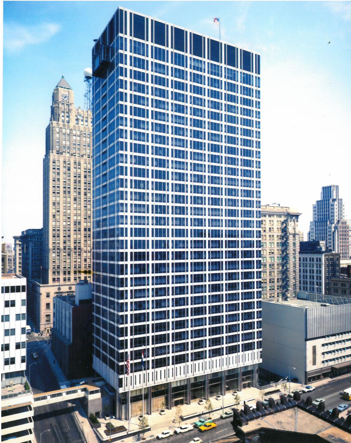
Figure 22. Historic photograph of Commerce Tower, c. 1965. Source: Wilborn Photography, Kansas City, Missouri.
