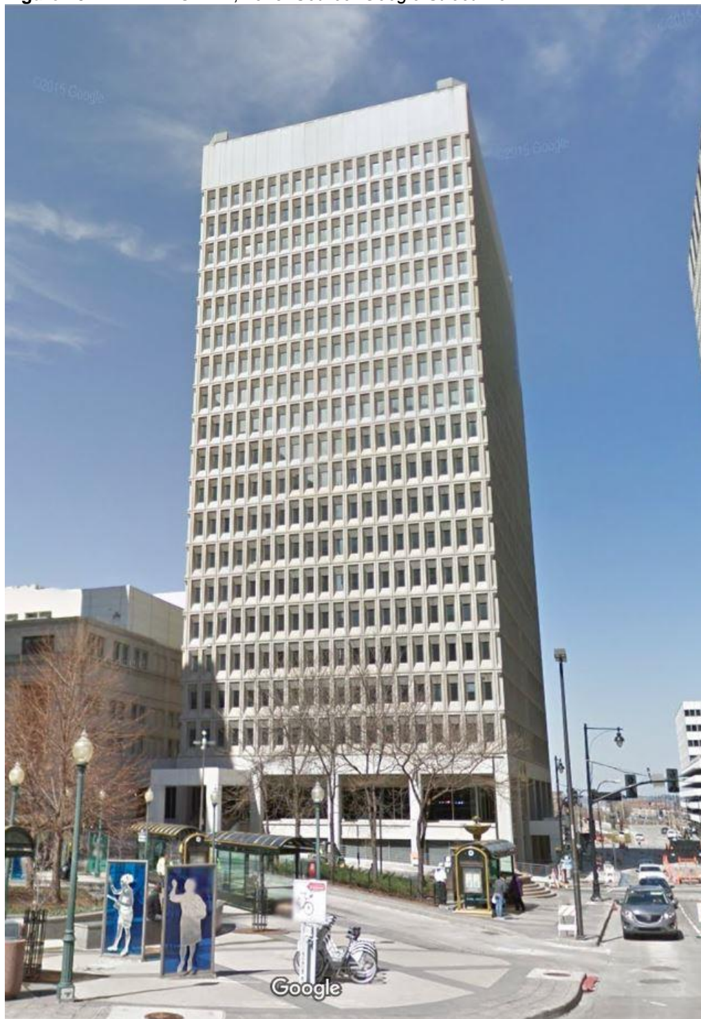
Figure 23. Ten Main Center, 2015. Source: Google Street View.
