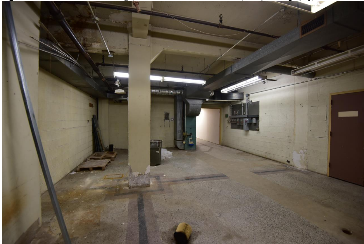
Figure 17: Basement of 1956 Garage, view west. Source: Brad Finch, f-stop Photography, 2015.
