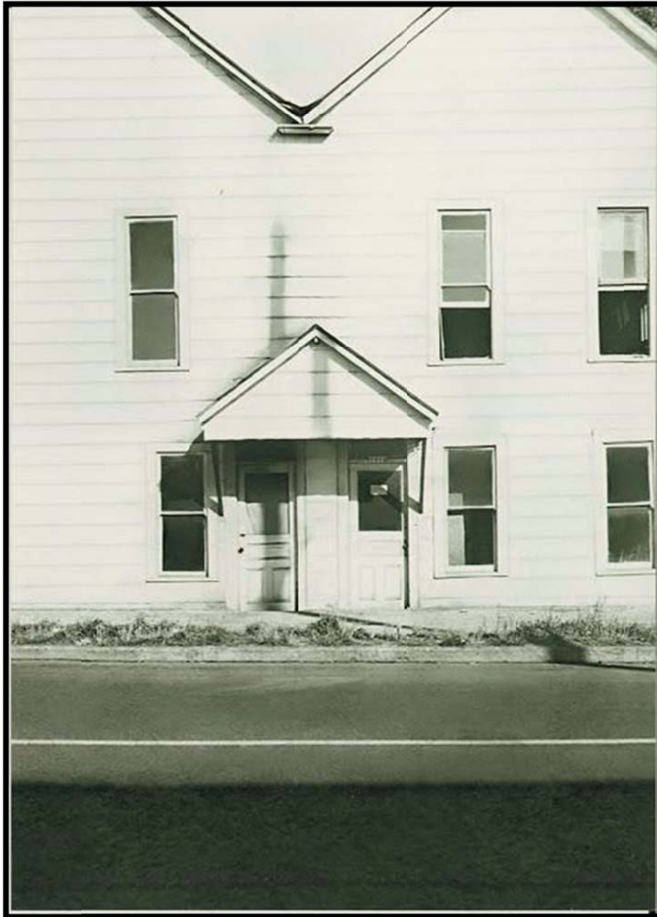
Figure 19: Vancouver Avenue First Baptist Church Photograph, 1947 1914 North Vancouver Avenue and Hancock Street Location
