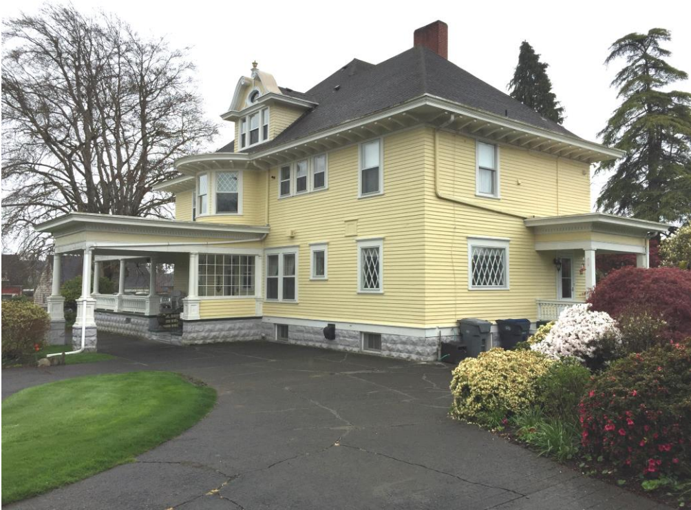
2 of 22. Northwest corner of Hulbert House showing back porch and porte cochere.
