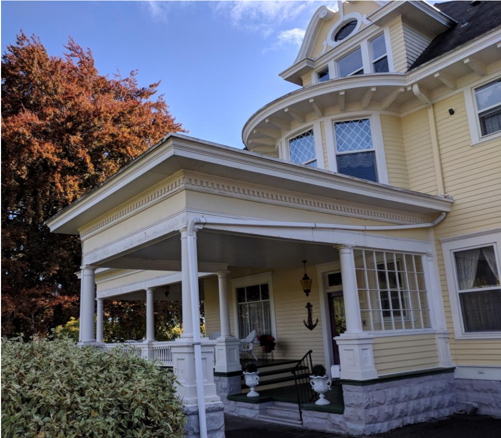
4 of 22. Detail of porte cochere.
