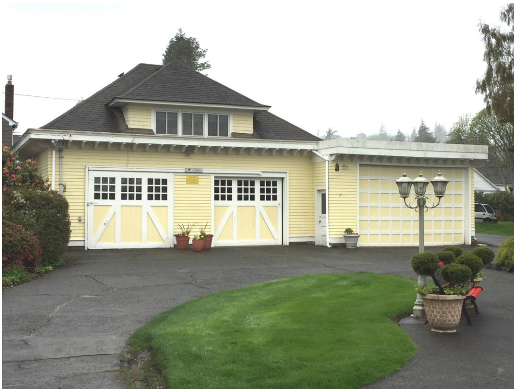
22 of 22. Carriage house/garage at rear of lot.
