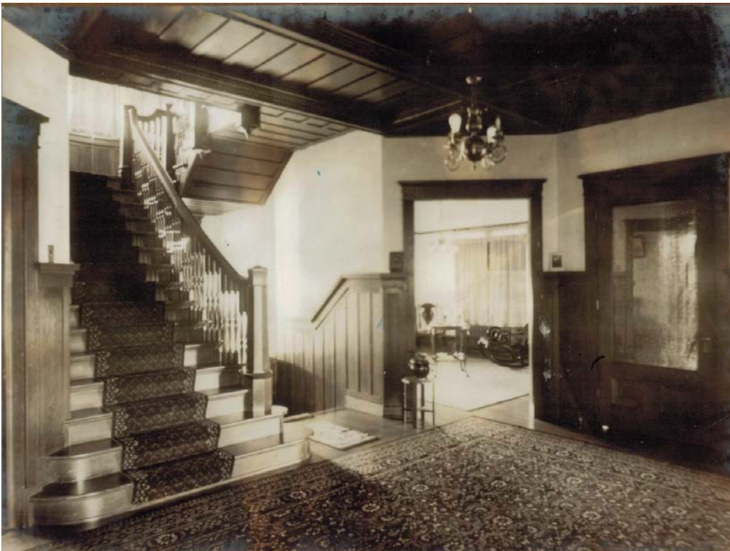
Entry foyer of Hulbert House looking towards second floor stairs – c. 1906 Photo courtesy of Jones Historical Photo Collection
