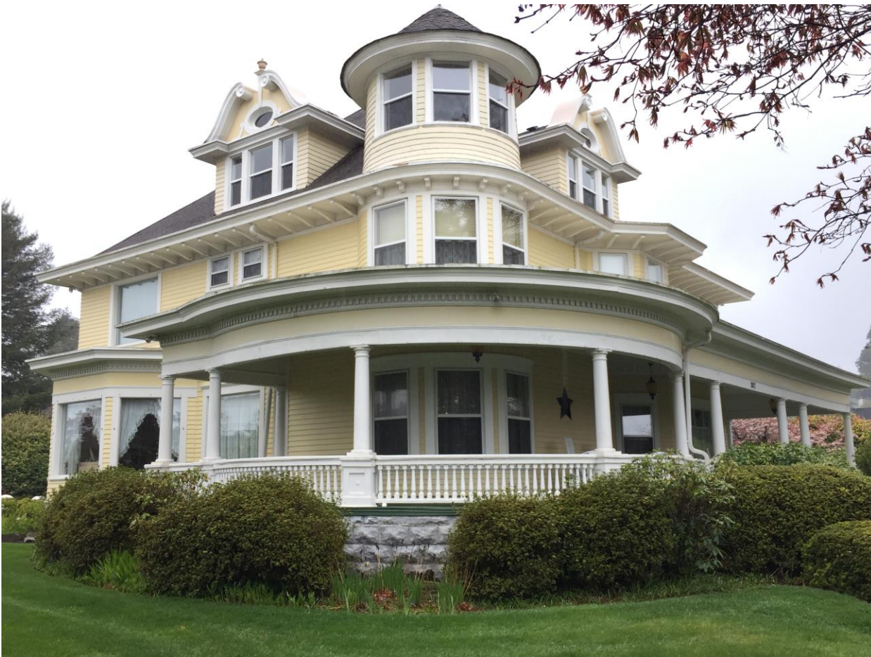
1 of 22. Southeast corner of Hulbert House showing wrap-around porch and turret.
