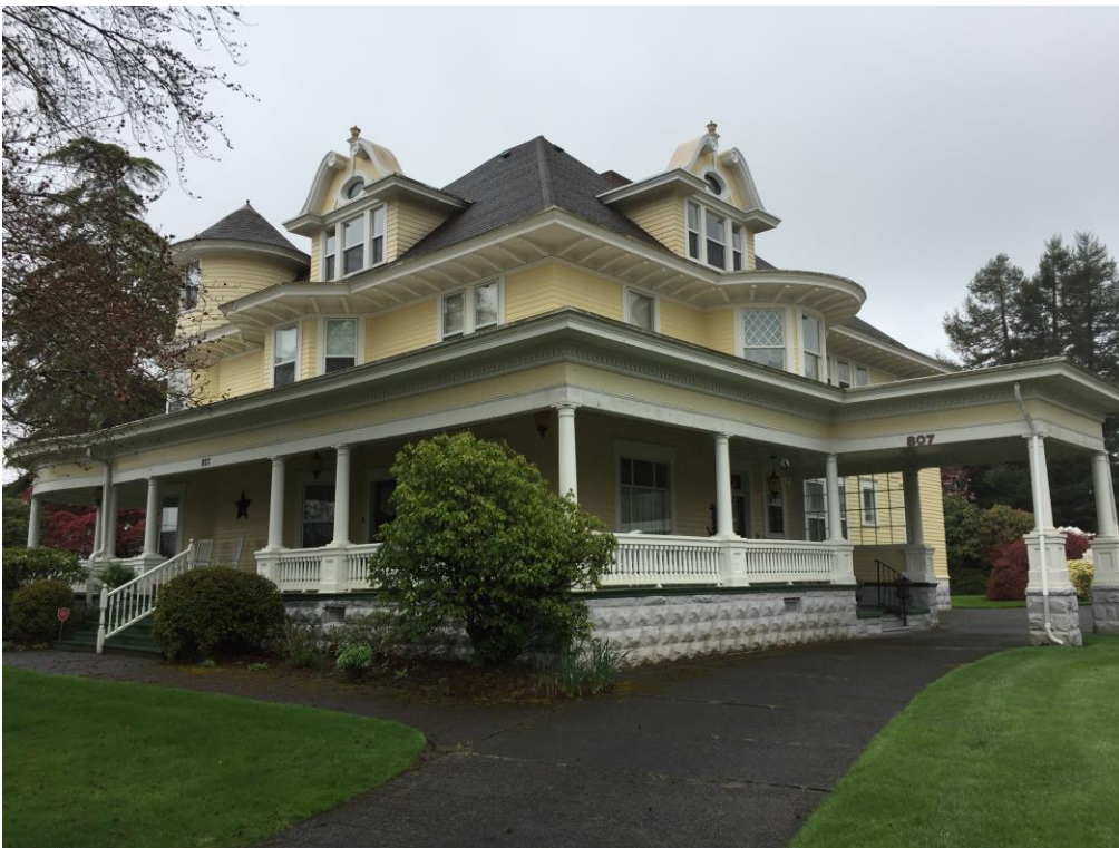
3 of 22. Northeast corner of Hulbert House showing wrap-around porch and porte cochere.
