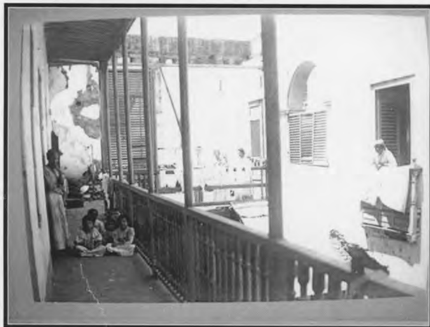
Figure 32. Interior patio of tenement house in Old San Juan, late 19 th - early 20 th centuries.
