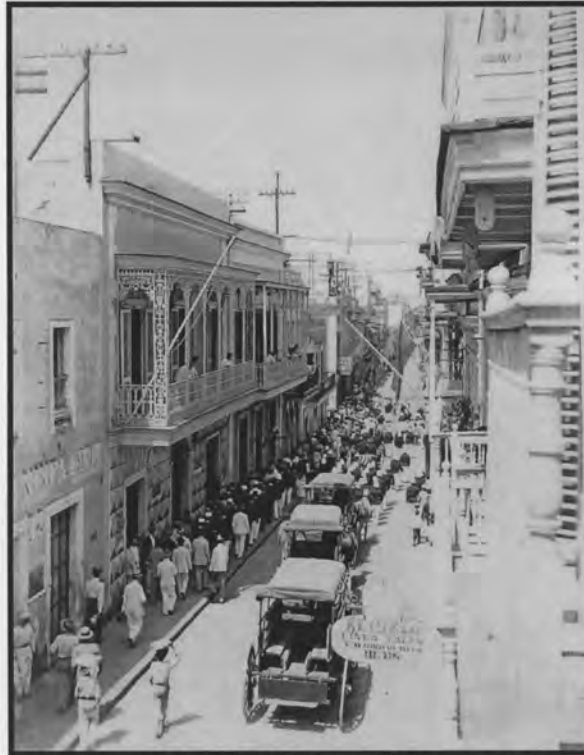
Figure 27. Street in the Old San Juan Historic District, c 1900. CP G Baynahr, Collection, PRSHPO.
