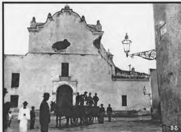
Figure 22. Iglesia de San José, showing damage caused by the May 11, 1898 bombardment. From: Crónica de la Guerra Hispano Americana en Puerto Rico , Ángel Rivero, 1922.
