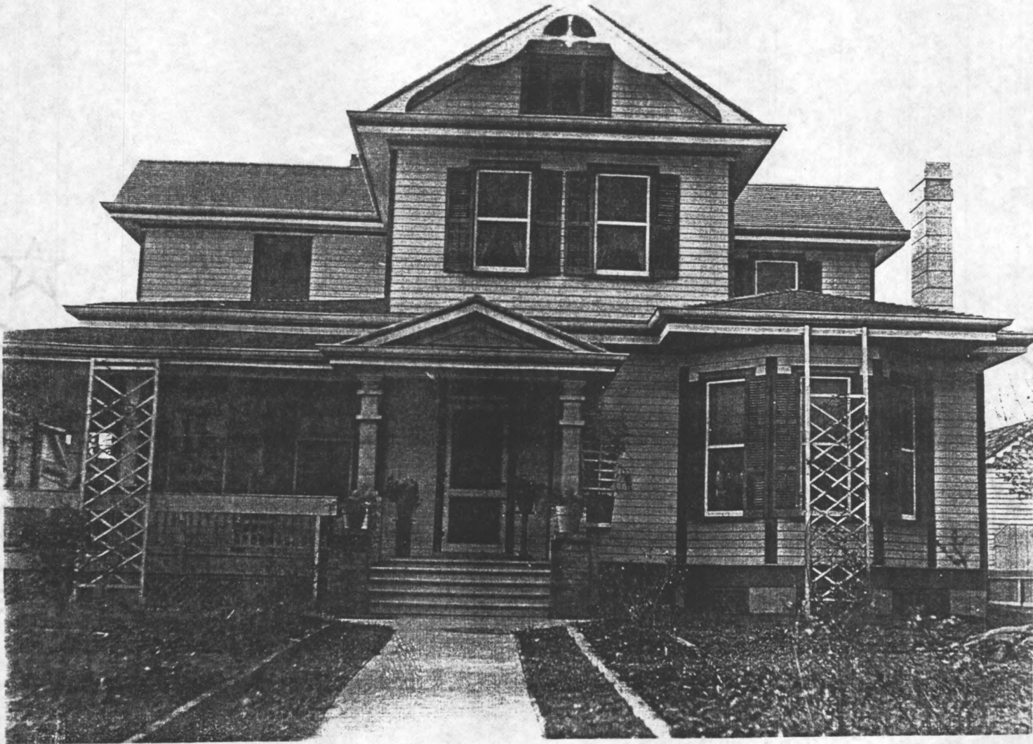
ORIGINAL APPEARANCE OF COOK HOUSE
