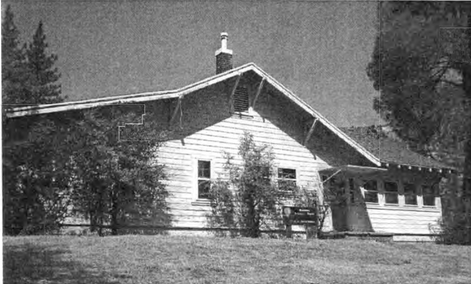
Example #1, Murchison House, El Portal, CA. Constructed by National Lead Company. Photographer: Jennifer Self, Architectural Historian Intern, Yosemite National Park Date: July 2009
