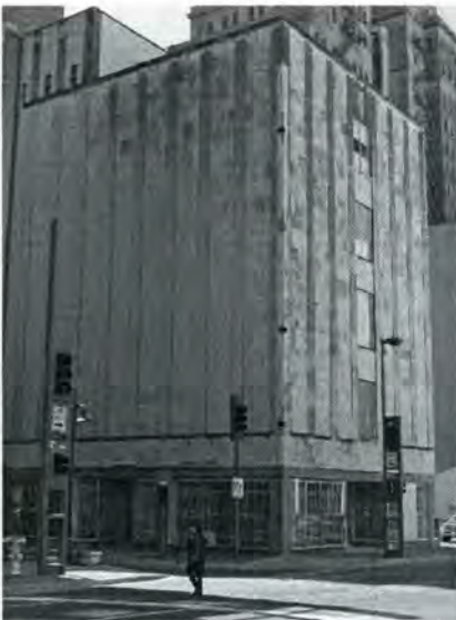
Original building, c. 1955 – 2005
