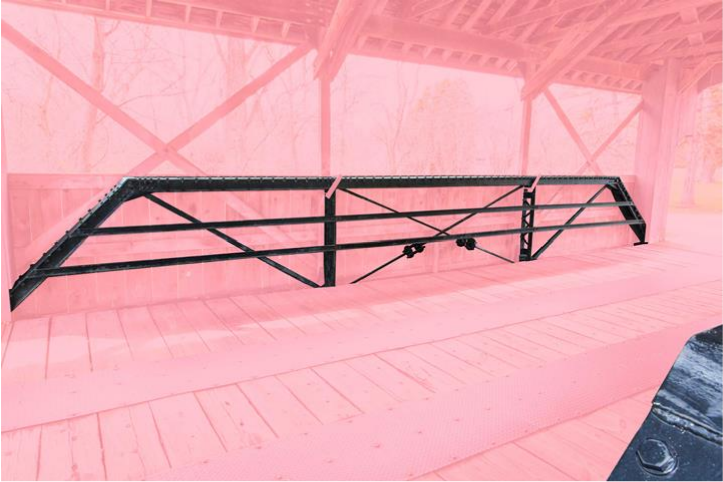
Figure 11: East Interior (non-historic elements shown in red) as seen from front of bridge.
