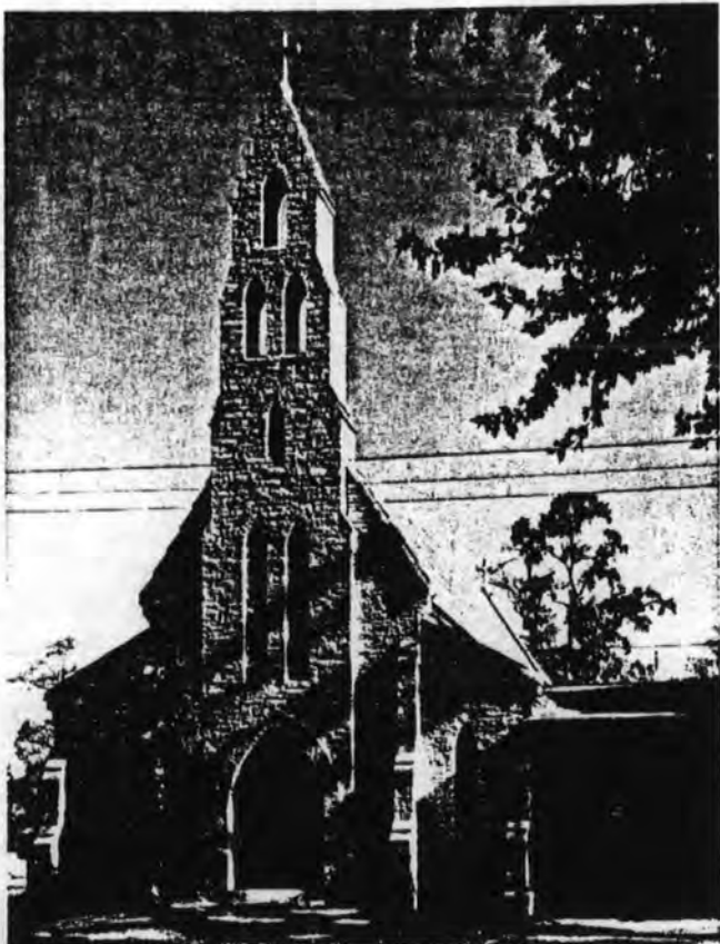
FIGURE 130. Richard Upjohn. Chapel of St. Mary the Virgin at Nashotah Episcopal Theological Seminary, Nashotah, Wis., west façade, 1859-60.
