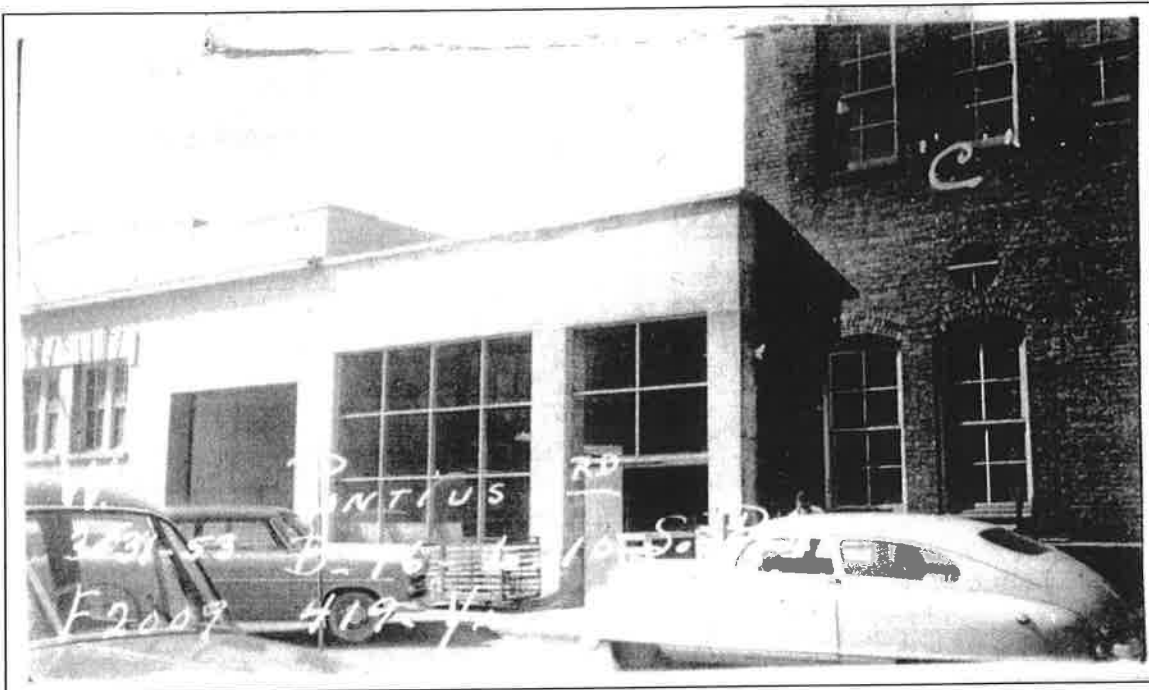
A 1953 property tax record photo of a one-story addition at the south end of the original building. This view is looking southwest and shows a portion of the original east facade (red brick) and the addition (concrete masonry unit). (Puget Sound Regional Archives)
