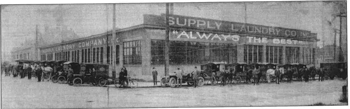
Looking southwest at the north and east facades of the Supply Laundry Building, ca. 1912. This view shows the earliest construction, before a second story addition. (Courtesy Tomlinson Linen Service)
