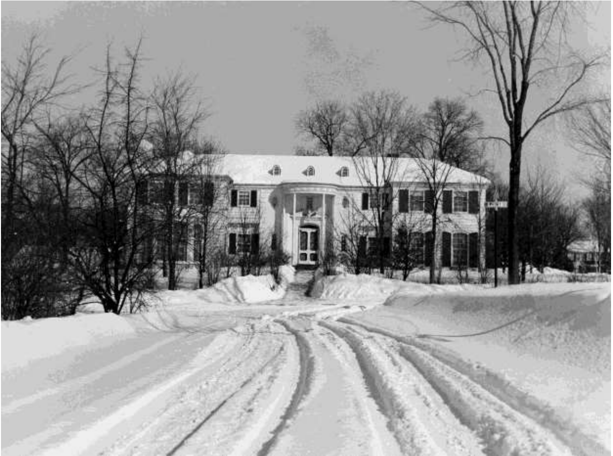
Figure 9: Main south Façade in winter. 1950. Courtesy of Patrick A. Martin.
