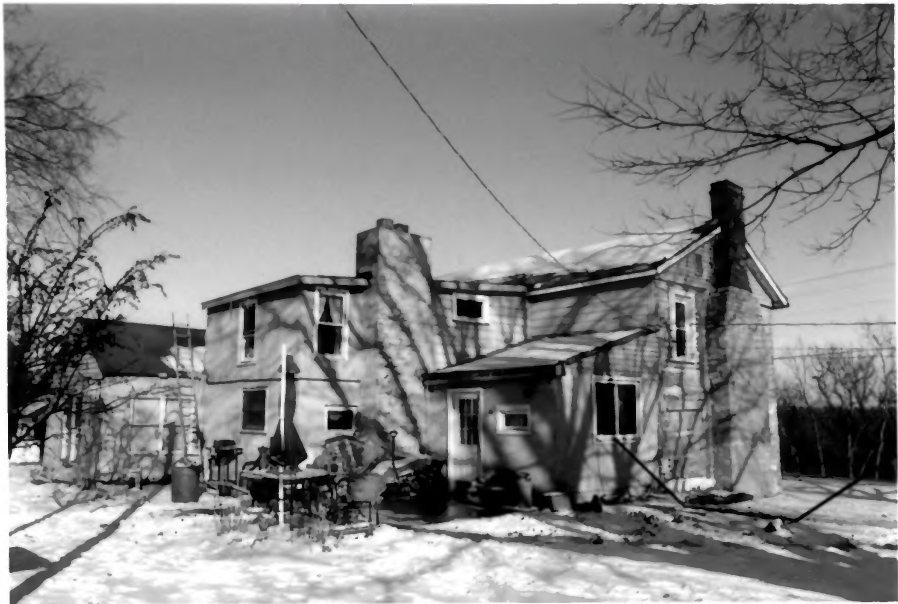
J. Q. A. Stephens House, Boone Co. KY 2
