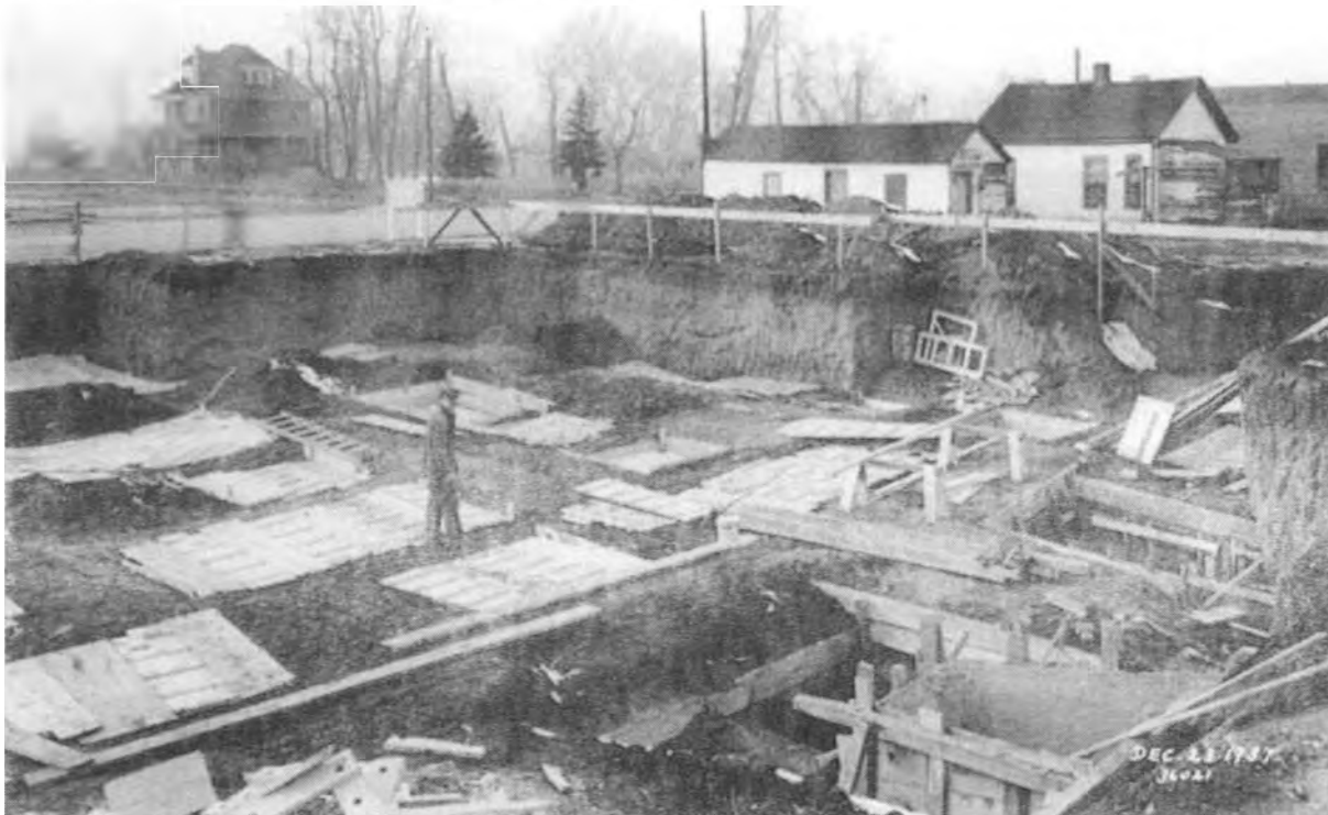
H4: Building concrete forms for the Englewood Post Office foundation, December 23, 1937. (Source: Denver Public Library, Western History Collection, Digital Photo Collection.)
