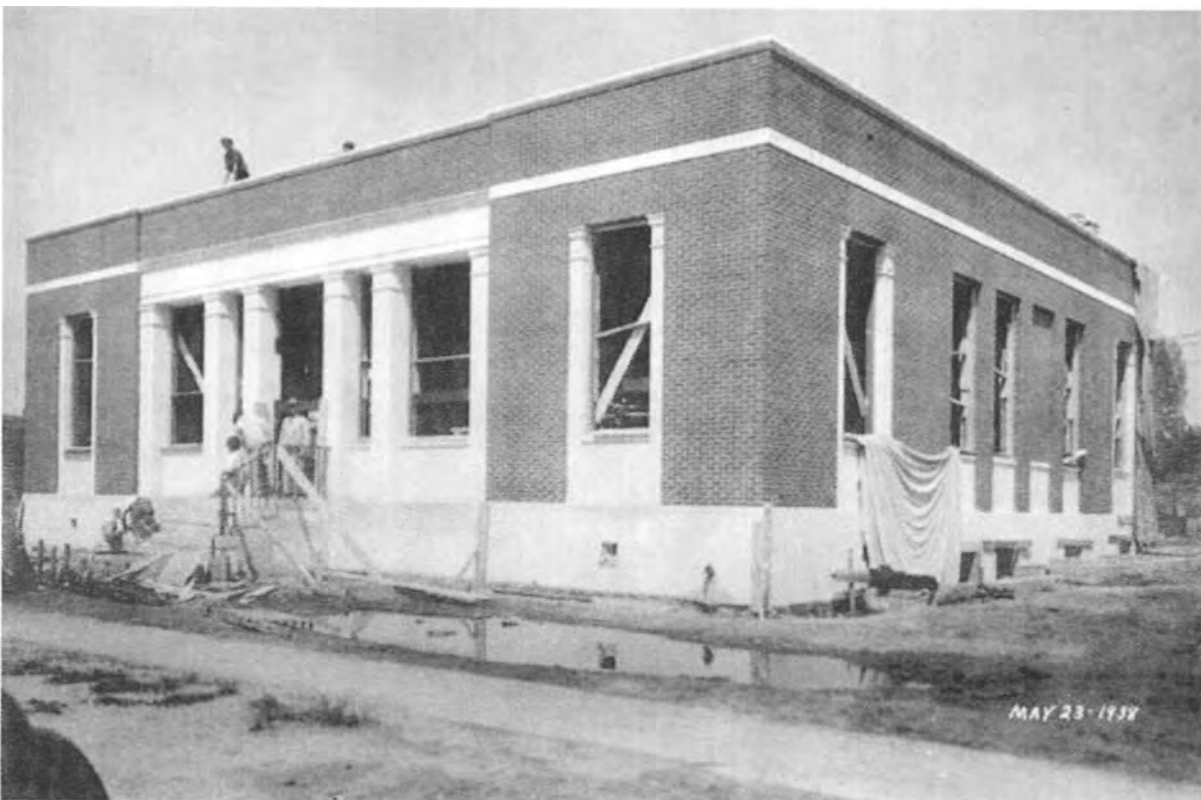
H6: The Englewood Post Office under construction, May 23, 1938. (Source: Denver Public Library, Western History Collection, Digital Photo Collection.)
