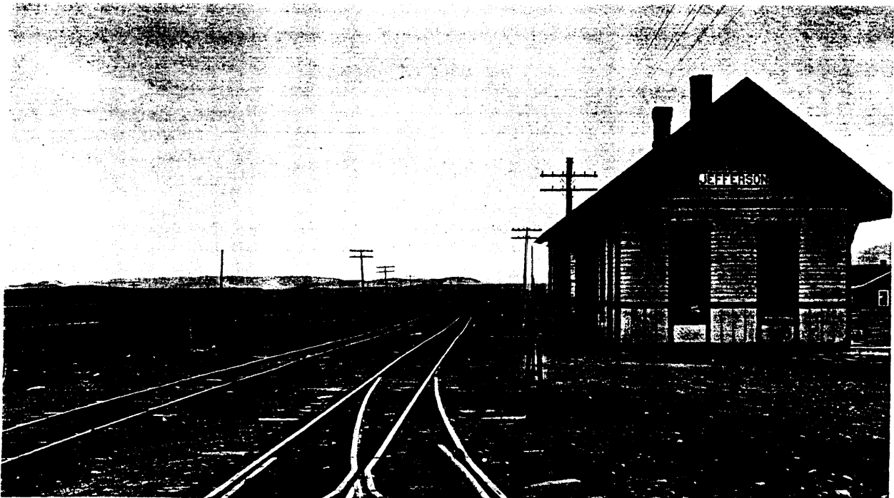
M. C. Poor photo, from David S. Digerness Collection.
